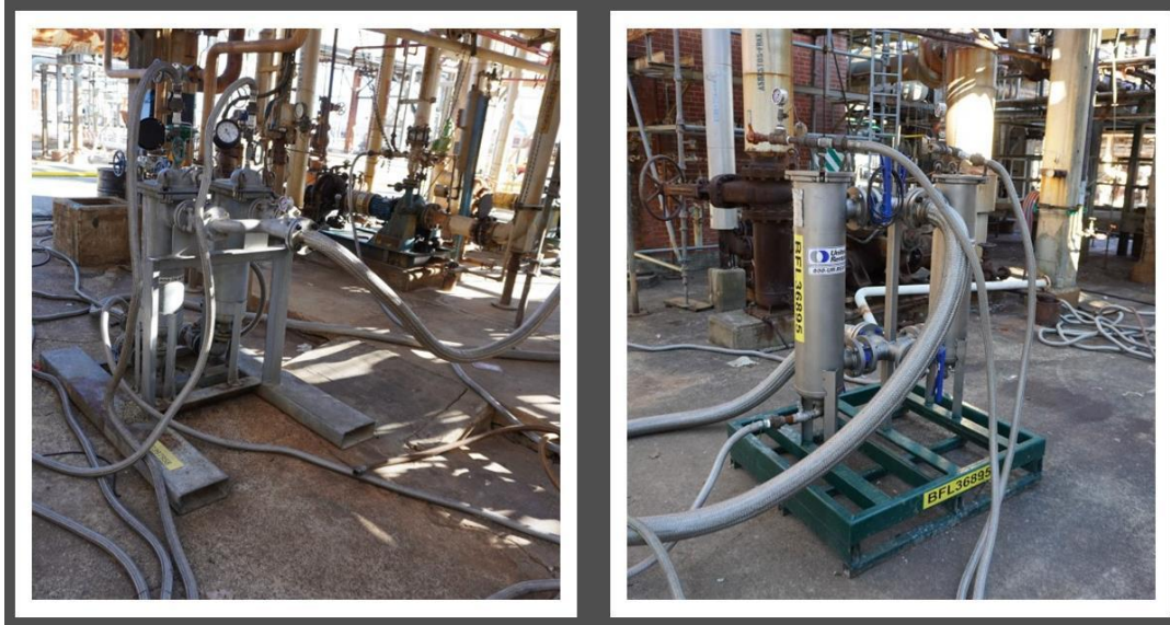
Figure 36. Photos of filter skids located elsewhere on the TPC PNO facility. (Credit: CSB)
