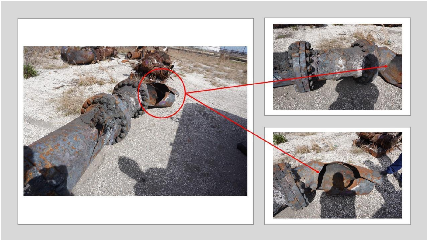
Figure 18. Photos of the recovered Final Fractionator A/B Primary Pump suction piping. (Credit: CSB)
