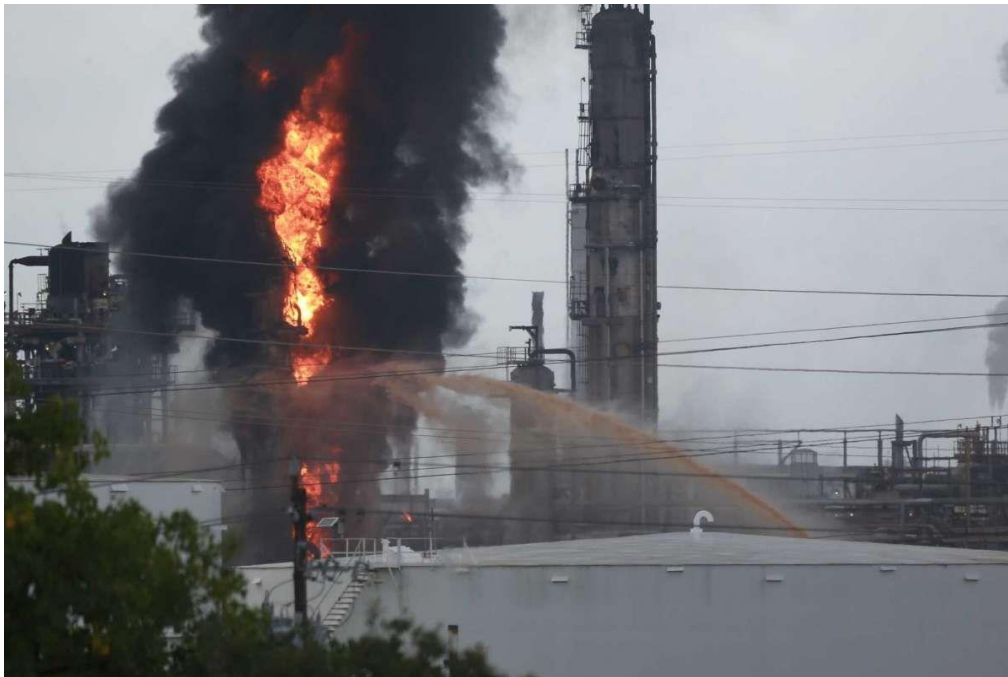
Figure 38. July 31, 2019, Baytown Incident. This picture shows the fire following the rupture of a section of 20-inch piping attributed to butadiene popcorn polymer. (Credit: Houston Chronicle [35]).
