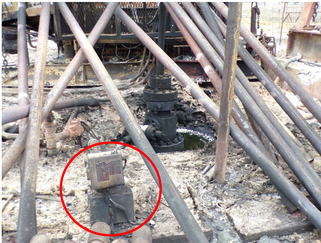
Figure 30. Hydraulic power pack (circled) location following the incident. (Credit: Chesapeake, annotation by CSB)
