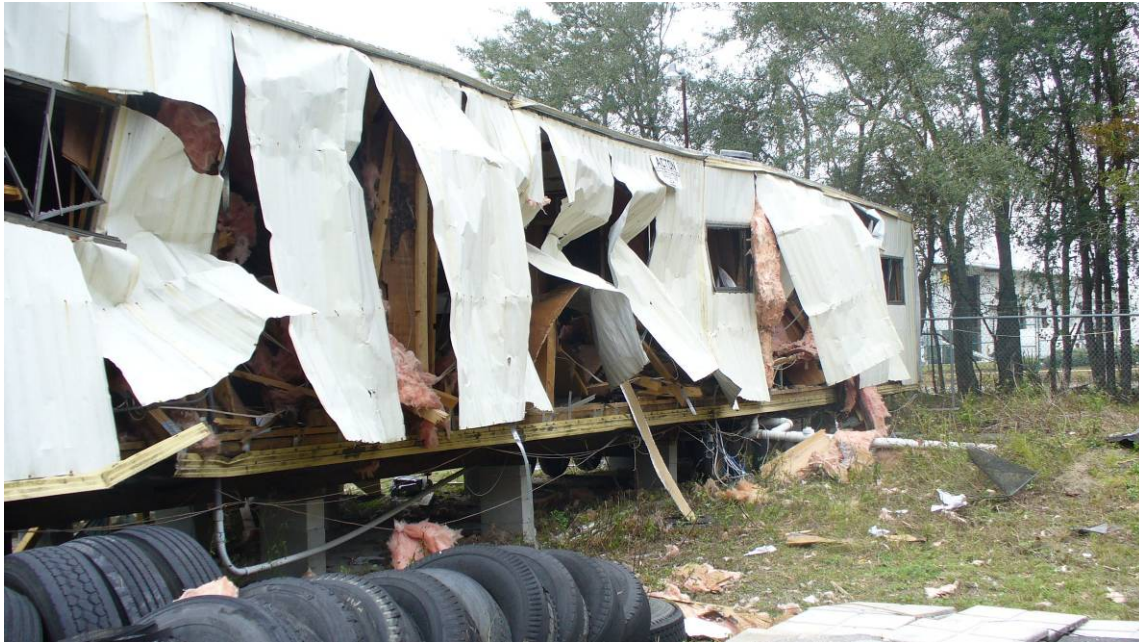
Figure 7. Trucking company trailer adjacent to T2.
