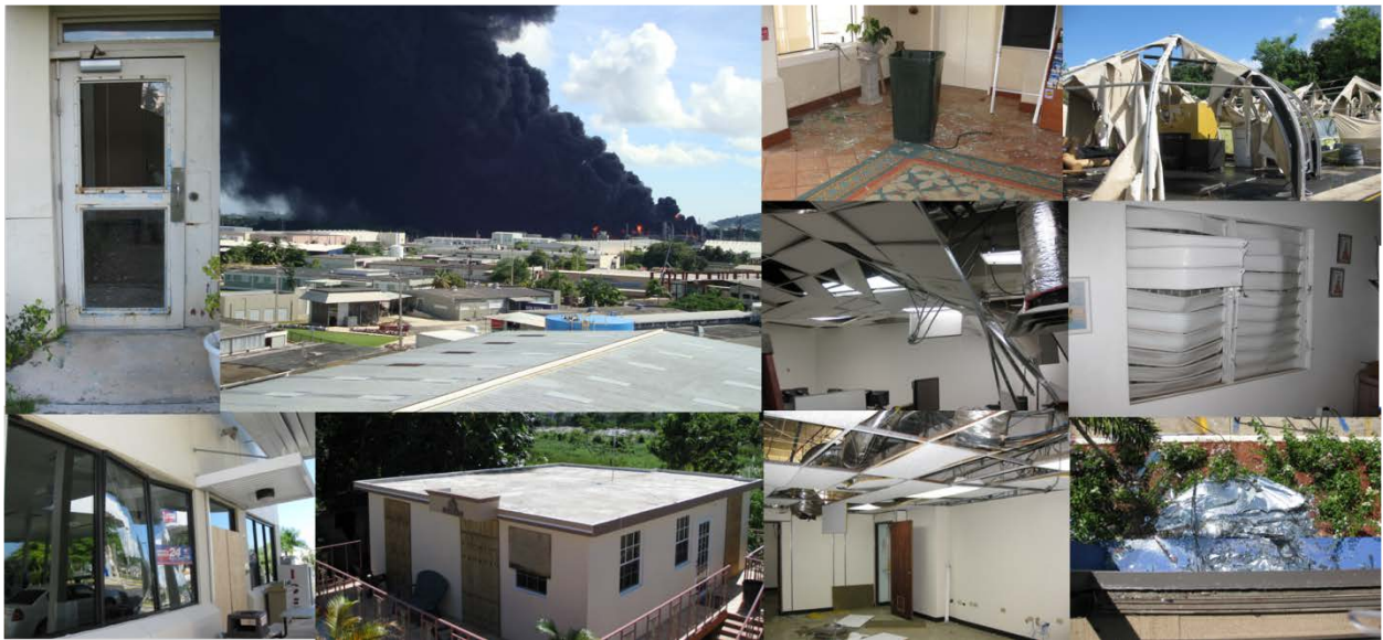
Figure 10: Community damage surrounding the CAPECO facility
