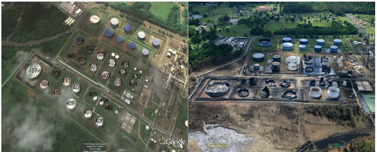
Figure 6: Impact of the explosion and multiple tank fires after the October 23, 2009 incident
