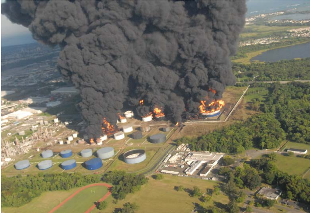
Figure 5: CAPECO multiple tank farm fire, October 23, 2009.
