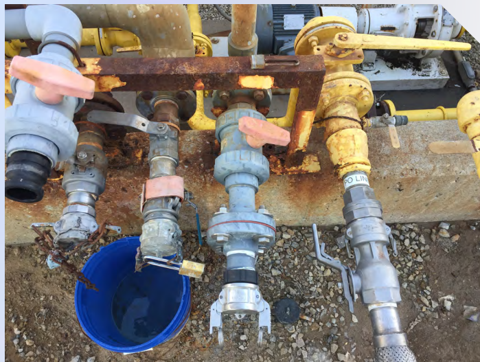
BEFORE: Old unloading portals (photo courtesy of CSB)
