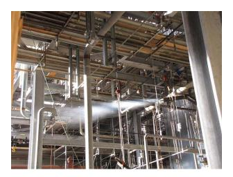
This cleaning practice is known within the natural gas power industry as a "gas blow." Industry personnel have indicated to CSB investigators that gas blows are a common practice during the commissioning of new or modified gas pipes at their facilities.
