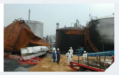
and caused significant off-site environmental impact. In June and July 2001, Motiva directed contractors to repair a catwalk that provided access to instrumentation on the roofs of six 415,000-gallon carbon steel sulfuric acid storage tanks. The catwalk had deteriorated due to acid vapors in the atmosphere around the tanks. The contractor employees worked this job over several days, cutting out damaged sections of the catwalk grating and welding down new sections.
