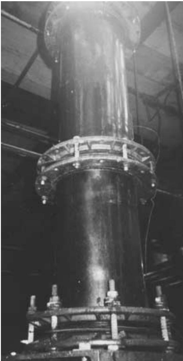
**Figure 8: Glass Section of 8-inch Line to Condenser**
