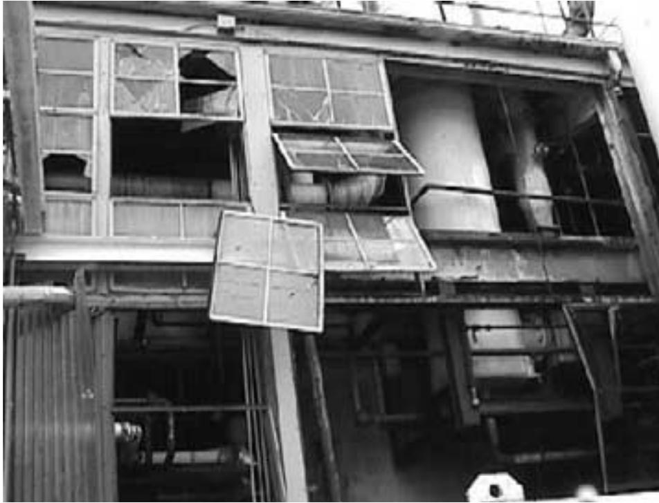
**Figure 13: Building 11's Blowout Panels and Window Frames**
