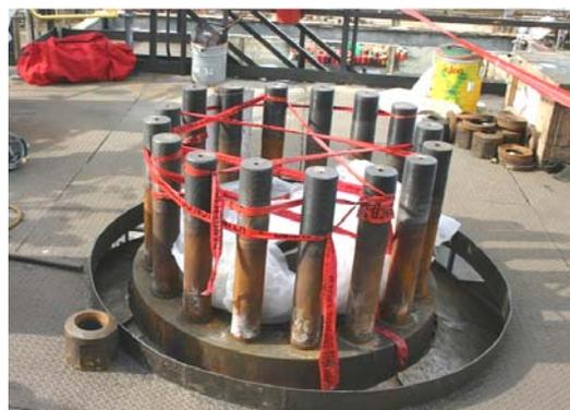
**Figure 1. Plastic sheet and plywood disk on R1 manway. Red "danger" tape on the studs alerted workers of the unsecured confined space access opening.**
