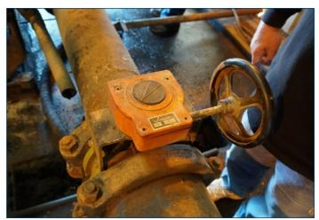
Figure 19. Position of the discharge (left) and suction (right) valves on Pump #1. (Credit: CSB)
