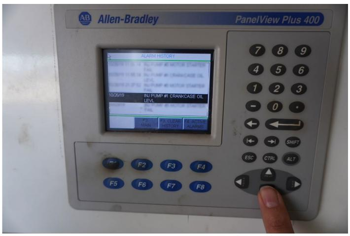
Figure 22. PLC screen displaying Pump #1 crankcase oil level alarm. (Credit: CSB)
