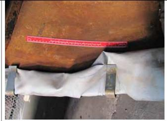
Fracture protection blankets and clip attachments
