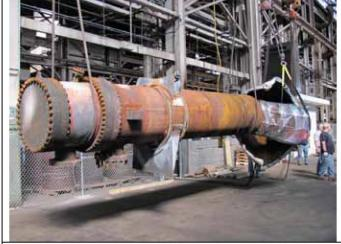
Main heat exchanger ready for wood saddle support insertion
