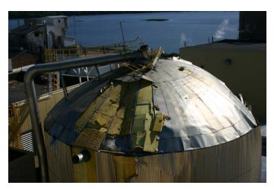
injured another. The CSB determined the explosion resulted from welding above an 80-foot-tall storage tank that contained highly flammable hydrogen gas – the product of bacterial decomposition of organic fiber waste inside the tank.
