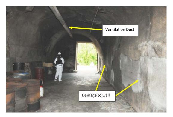
Figure 15. Damage to the magazine wall
