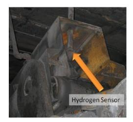
and press feed belt conveyor system would activate the deluge of water if readings reached a designated alarm point (illustrated in Figure 16). Operators also could manually activate the deluge system by turning a valve located in the blending and press room.
