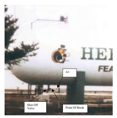
Figure 4. Liquid Line Shut-Off Valve and Point of Break
