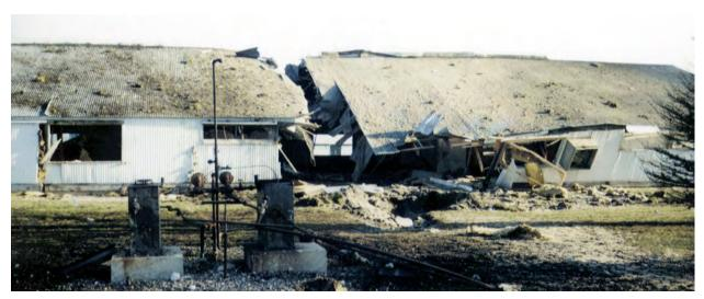
Figure 12. Damage to Turkey Barn (1g) Caused by Impact of Large Tank Fragment
