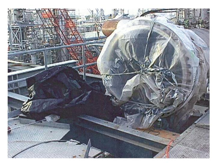
Figure 2. Clear Plastic Sheet Covering One Of The Pipe Openings
