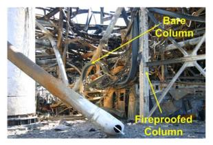
Figure 7. Fireproofed and bare steel support columns.
