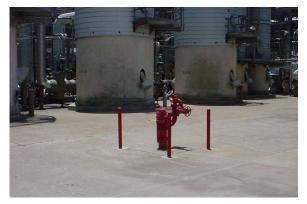
Figure 9. Protection of fire fighting equipment.
