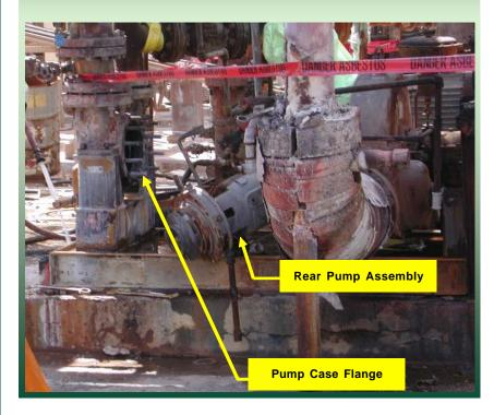
The plant operator placed tags and locks on the suction and discharge valves to prevent inadvertent opening and to indicate that the valves had been closed. The mechanic specialist then placed tags and locks on the suction and discharge valves. When the mechanic returned, the mechanic specialist told him that the valves had been closed, secured, tagged, and locked per the facility's LOTO procedure and that they could remove the pump.
