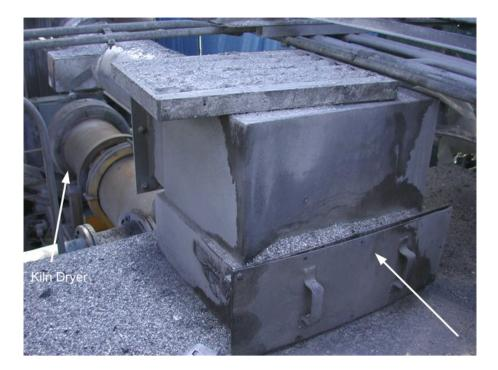
Figure 19. Wet chip hopper target box, with bulged access door (arrow).
