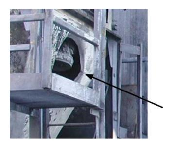
Figure 23. Air inlet (arrow) on the south side of the dust collector.
