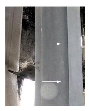
Figure 25 Beam slightly deflected by drop box impact. Arrows on either side of the point of impact show the direction of bending
