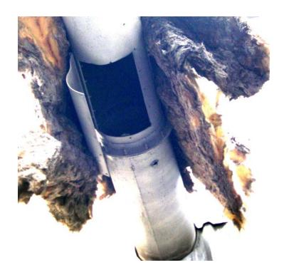
Figure 28. Cleanout door blown open on duct from furnace 5 fume hood to fume separator. Insulation from the roof rests on the duct (Figure 4 shows the location of this duct in the building).
