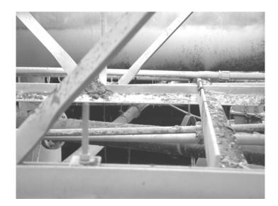
Figure 34. Dust accumulation on roof trusses.
