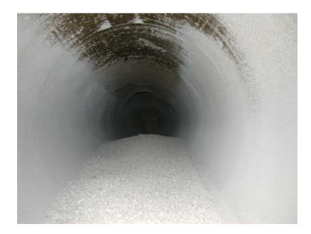
Figure 26. Interior of main duct between the chip equipment and the drop box with significant dust and chip accumulation.
