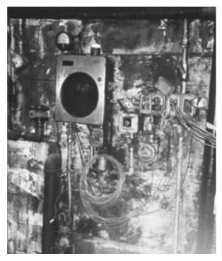
Figure 5: Temperature Chart and Digital Display
