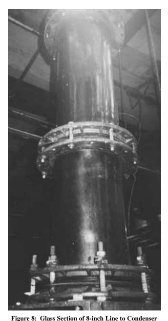
The 8-inch line to the condenser had a glass section above the kettle head in which turbulent, refluxing vapor could be seen in Yellow 96 batch 32.
