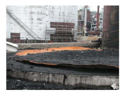
Figure 8. Floor of tank 393 showing uplift due to internal deflagration (before separation of shell).
