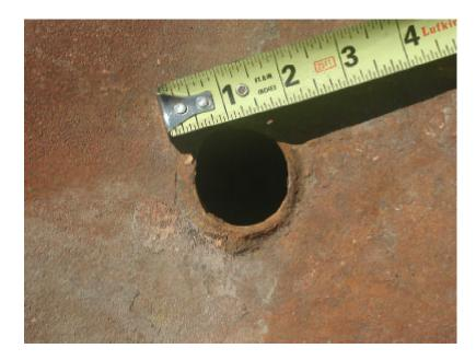
Figure 6. Hole in roof of tank 393 through which temporary hose was inserted.
