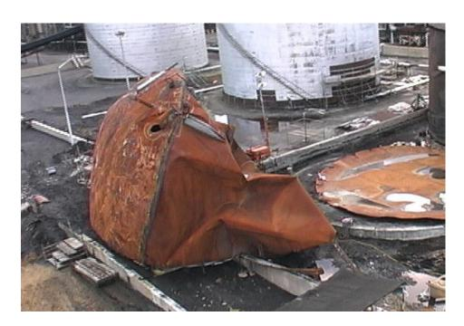
Figure 2. Tank 393, collapsed at northeast corner of storage tank dike. (Note floor of tank 393 to the right of tank shell.)
