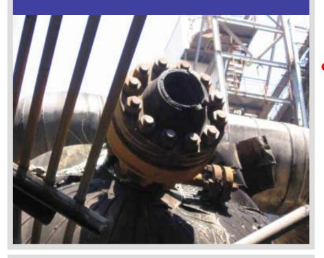
Figure 3. Ruptured 8-inch pipe elbow on heat exchanger A outlet.
