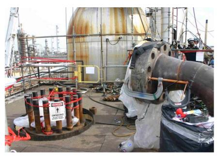
This Case Study describes the Valero Delaware City refinery asphyxiation death of two contractor employees who were preparing to reassemble a pipe on a pressure vessel while it was being purged with nitrogen. The first worker, in an attempt to retrieve a roll of tape from inside the vessel, was overcome by nitrogen, collapsed in the vessel, and died. His co-worker, the crew foreman, was asphyxiated while attempting to rescue him.
