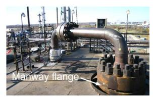
Figure 2. Pipe assembly connects 12-inch diameter process pipe to the reactor top manway (photo taken after the incident).
