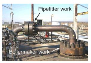
Figure 9. Pipefitters assembled 12-inch pipe flange, boilermakers assembled 24-inch manway flange.
