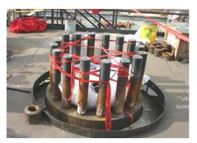
Figure 1. Plastic sheet and plywood disk on R1 manway. Red "danger" tape on the studs alerted workers of the unsecured confined space access opening.
