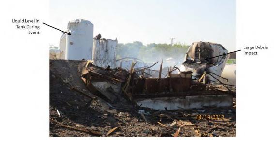
Figure 16. Liquid Fertilizer Tank Damage (Source: CSB)
