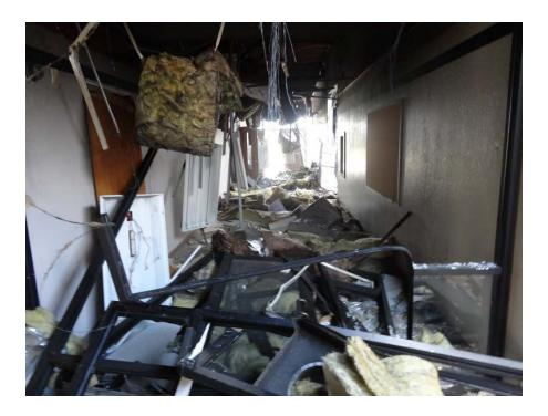
Figure 24. WIS North Hallway, Looking Toward Northeast Exit Door (Source: ABS Consulting)
