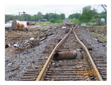
Figure 18. Damaged Railroad Tracks Adjacent to WFC Facility (Source: CSB)
