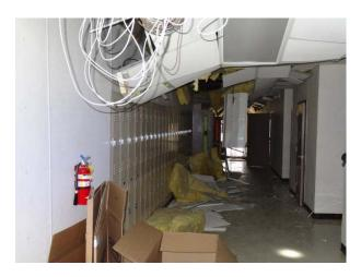
Figure 32. Classroom Annex Interior Hallway and Ceiling Damage at WMS (Source: ABS Consulting)
