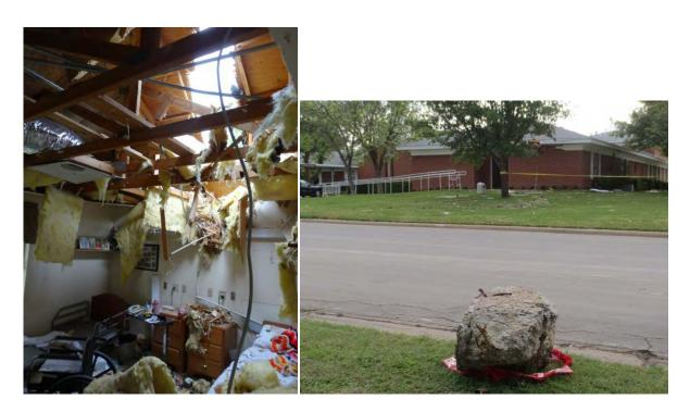
Figure 35. Crater and Debris (left) from Fragment (right) of WFC Facility Foundation that Impacted West Rest Haven (Source: ABS Consulting)
