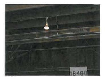
Figure 53. Exposed 440-Volt Electrical Wiring Identified in 2007 Survey (Source: Triangle Insurance Company)
