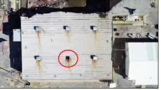
Roof opening at broken duct, Low Bay roof north of High Bay tower (Atlas 9/29/2020)
