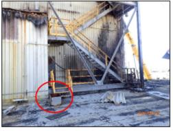
Roof-top ductwork torn away, at two roof areas adjacent to Low Bay
