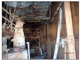
3<sup>rd</sup> floor level from north stair, showing heatdeformed columns & bracing (Atlas, 9/29/2020)
