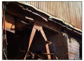
Ground floor level looking east, showing heatdeformed brace & spandrel (Atlas, 9/29/2020)
