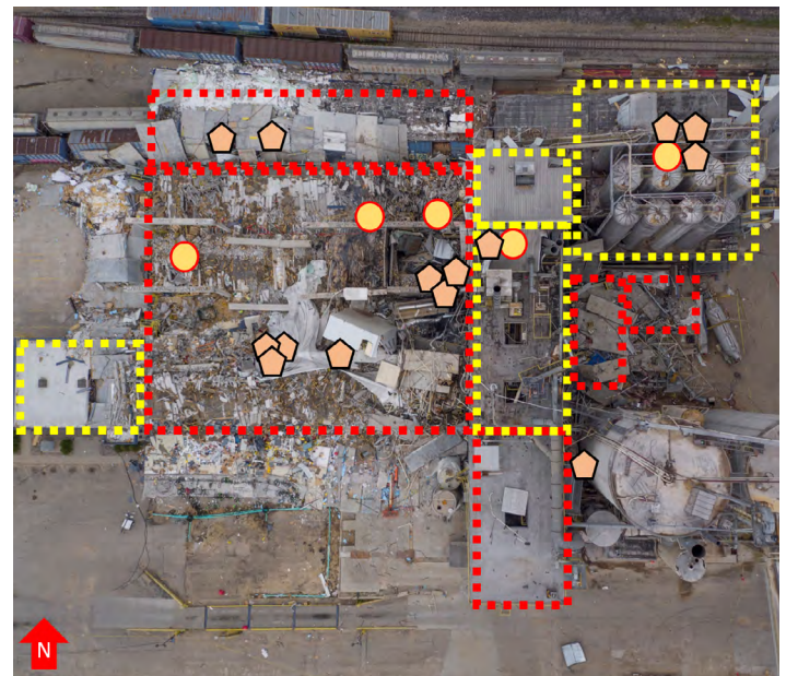
Figure 3. This visual depicts the approximate locations of workers inside the Didion facility at the time of the incident. Circles represent workers who sustained fatal injuries, and the pentagons represent injured workers. Red dotted outlines indicate buildings that had completely collapsed or were severely damaged by the explosions on May 31, 2017. Yellow outlines indicate buildings that were accessible to investigators, but sustained severe damage. B Mill was partially accessible.
