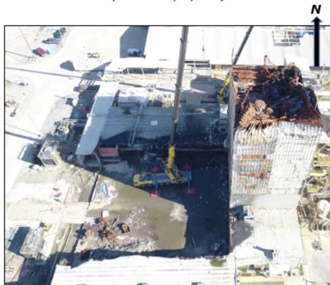
Open roof duct at 30-day Warehouse, just south of Low Bay (Atlas UAV 9/30/2020)
