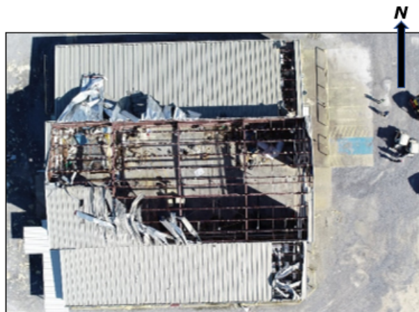
A-Z Building (Atlas UAV, 9/30/2020)
