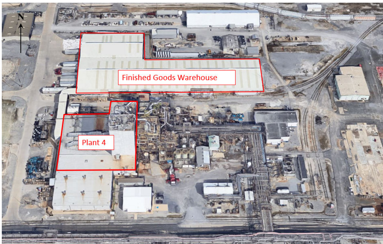
Figure 1. Overhead view of a portion of the Bio-Lab facility with red denoting buildings involved in the incident. (Credit: Google Earth, annotations by U.S. Chemical Safety and Hazard Investigation Board (CSB))
