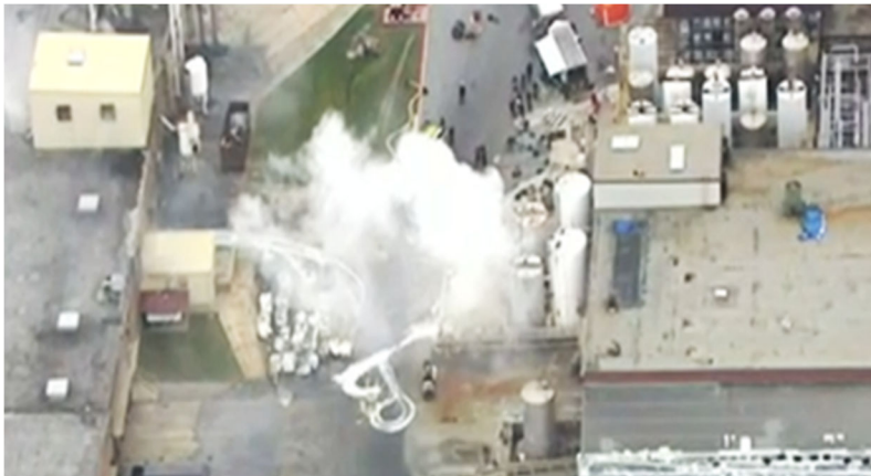
Figure 27. TCCA decomposition products, including chlorine, releasing from the Bio-Lab Conyers facility on September 14. (Credit: WSB-TV Channel 2 Atlanta)
