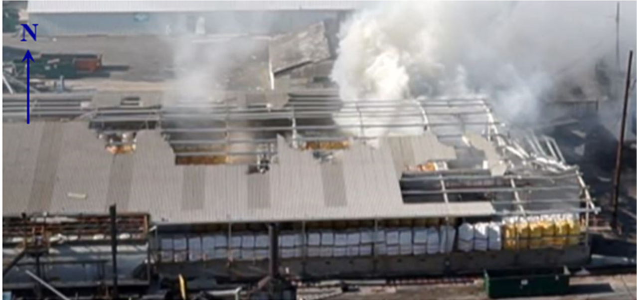
Figure 13. Damaged Finished Goods Warehouse roof emitting white fumes. (Credit: Bio-Lab)
