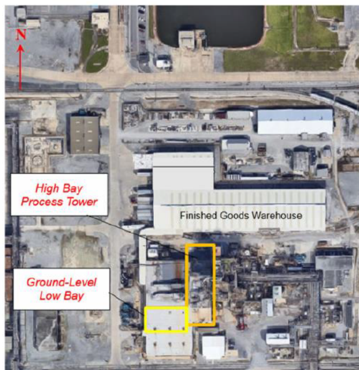
Figure 1: Plant 4 and Finished Goods Warehouse
