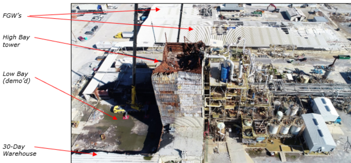
Overview, looking north (Atlas UAV, 9/30/2020)
