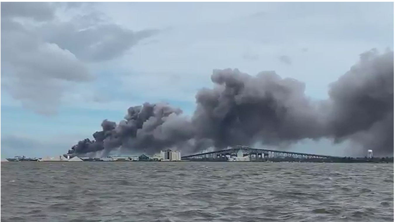
Figure 8. Photo of plume from TCCA decomposition in Bio-Lab Plant 4 approaching the Calcasieu River Bridge near the facility. (Credit: CBS 4WWL [22])
