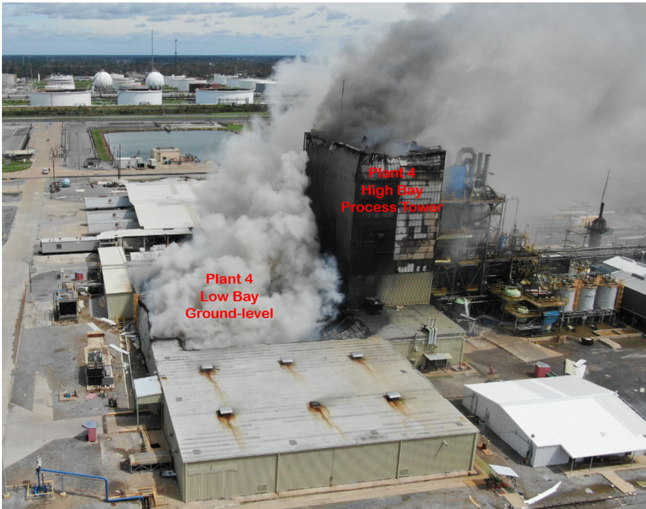
Figure 9. Decomposing TCCA in Plant 4 on August 27, 2020. (Credit: Louisiana State Police, annotations by CSB)
