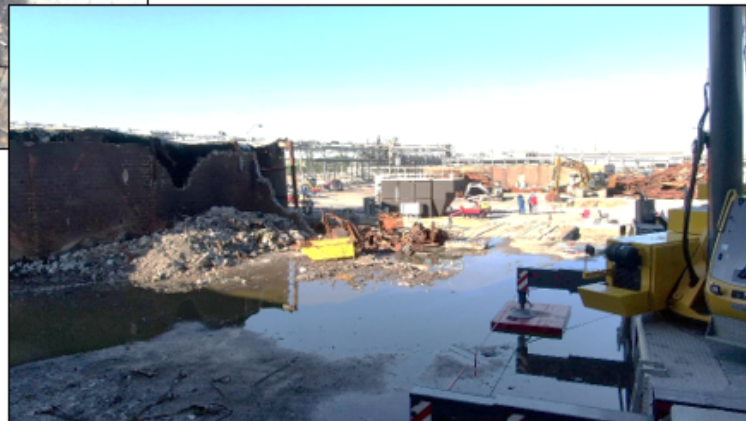
View looking west (Atlas UAV, 9/30/2020)
