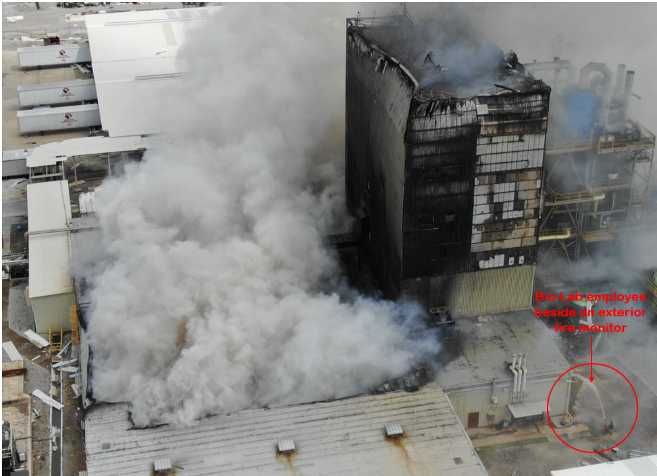
Figure 11. Available water pressure at an exterior fire monitor near Plant 4. (Credit: Louisiana State Police, annotations by CSB)
