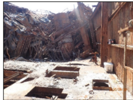
4 th floor level, from north stair (Atlas 9/29/2020)
