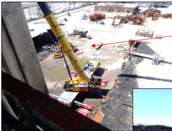
View from High Bay stair, looking SW (Atlas, 9/29/2020)
