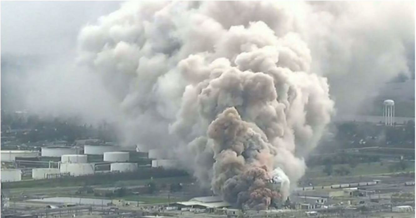
Figure 7. Photo of TCCA decomposition gases, including toxic chlorine, released from Bio-Lab Plant 4 after the building was severely damaged during Hurricane Laura and rainwater contacted the stored TCCA. (Credit: The Associated Press [21])
