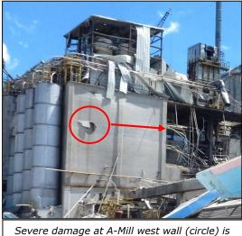
Severe damage at A-Mill west wall (circle) is at same elevation as fractured airshaft at 4B (arrow). (photo by Atlas)
