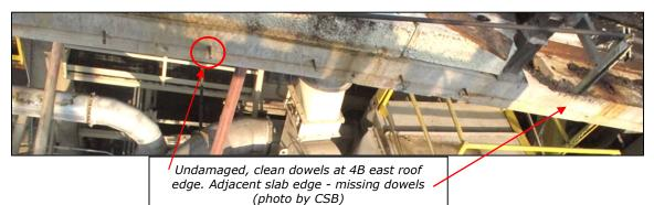
In post-blast photos, the exposed dowels show no signs of yielding. The exposed bars are relatively clean of epoxy residue or concrete debris. Photos show no pattern of concrete damage at the panels along the lines of the dowel holes, either at the panels that fell off 4B, or at the 1B-3B panels that bulged outward from the building.
