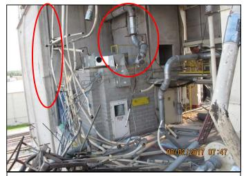
NW corner of 4B, showing fractured airshaft walls (circle at right). Note bulged and cracked wall at A-Mill, just a few feet away (circle at left). (photo by CSB)
