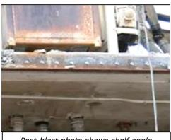
Post-blast photo shows shelf angle intact at B-Mill floor slab; no signs of broken welds. (photo by CSB)
