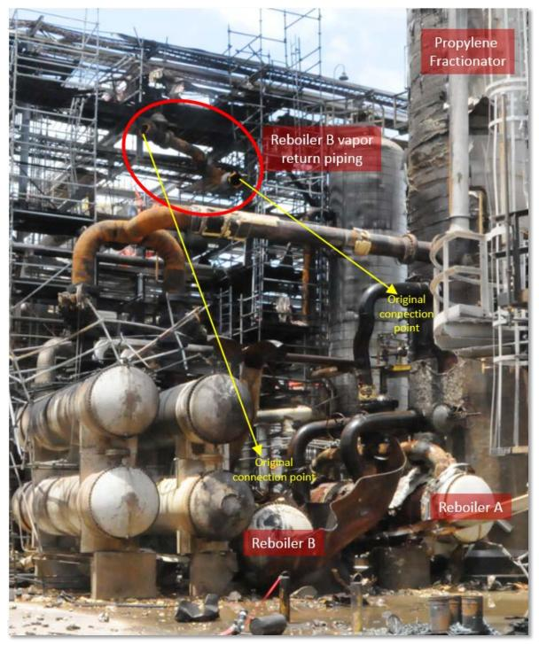
Post-incident photo of the propylene fractionator reboilers and surrounding area. The Reboiler B vapor return piping can be seen overhead in the pipe rack (red circle). The approximate original configuration of the piping and equipment is shown in Figure 9 and Figure 14.
