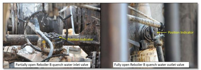
Post-incident, the Reboiler B quench water inlet ball valve was found partially open (left), and the Reboiler B quench water outlet ball valve was found fully open (right). When the position indicator is parallel to the pipe, the valve is open; when the position indicator is perpendicular to the pipe, the valve is closed.
