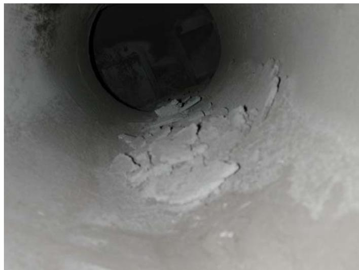
Figure 29. Interior of fume duct to fume separator (near the cleanout door.)
