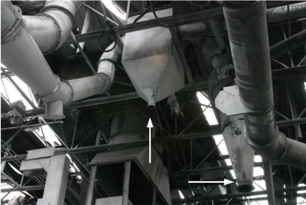
Figure 31. Unused spark box and cyclone, with openings (see arrows) where sparks could be pulled into the dust stream by the airflow.
