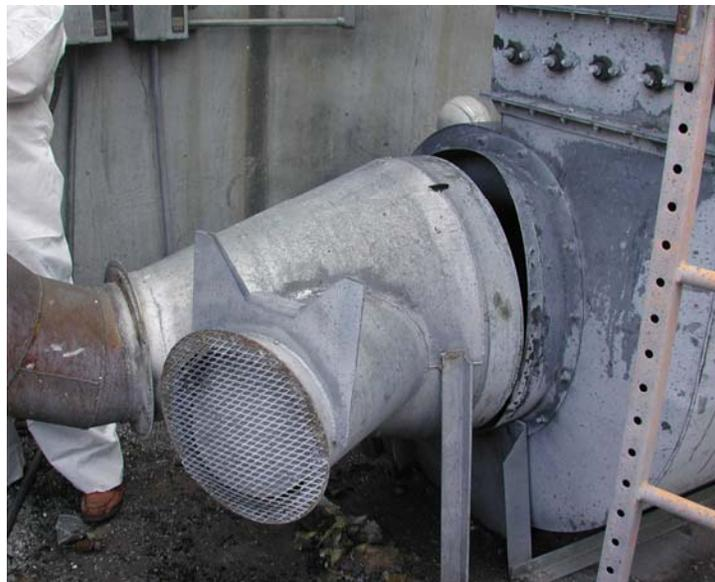
Figure 27. Fume hood exhaust fan cover damaged by overpressure.
