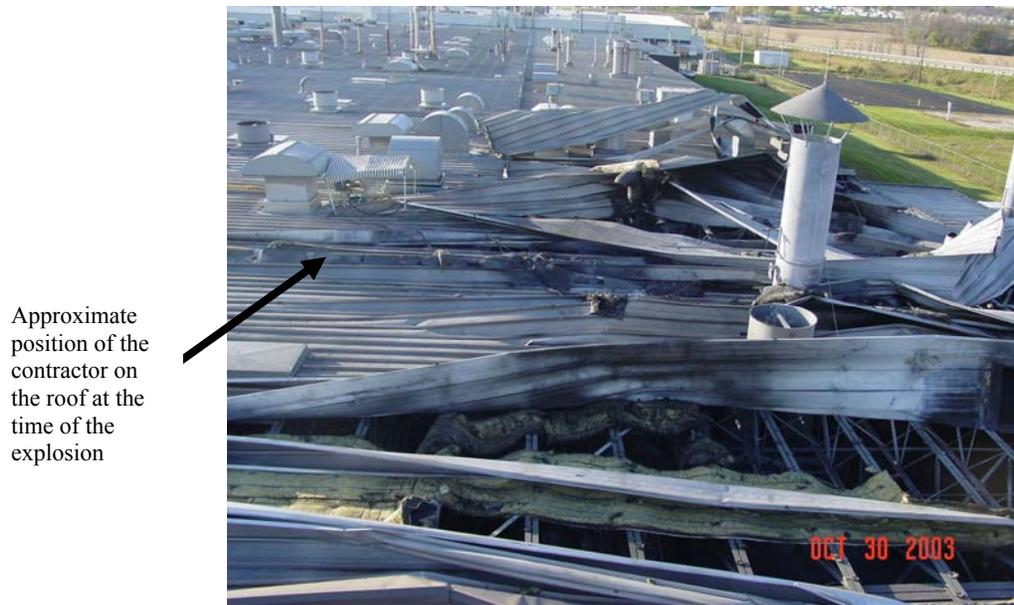
Figure 13. Damaged roof above furnace 5.
