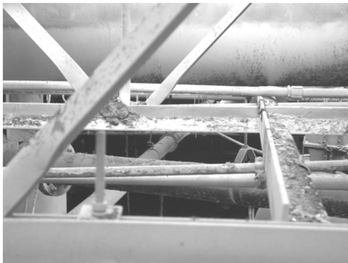
Figure 34. Dust accumulation on roof trusses.
