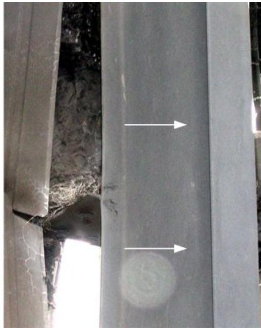
Figure 25 Beam slightly deflected by drop box impact. Arrows on either side of the point of impact show the direction of bending
