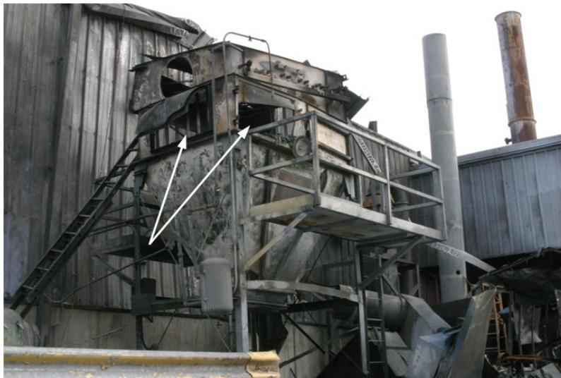
Figure 21. Explosion vent panel and maintenance door (arrows) blown out on dust collector.
