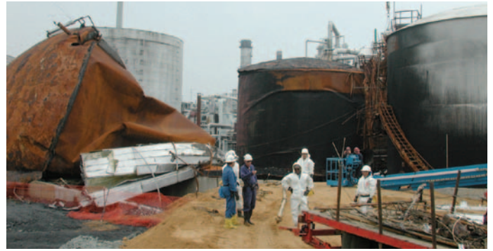
A view of the flammable storage tank involved in the accident at the Motiva Refinery.
