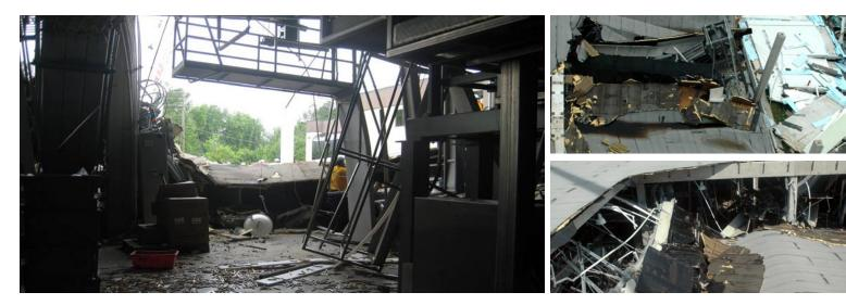
Interior of ConAgra facility following structural collapse.
