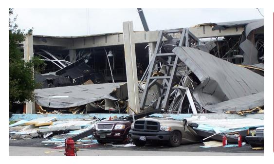
The ConAgra Slim Jim plant in Garner, North Carolina, where unsafe gas purging caused an explosion in June 2009 that killed three workers and sent 71 to the hospital.
