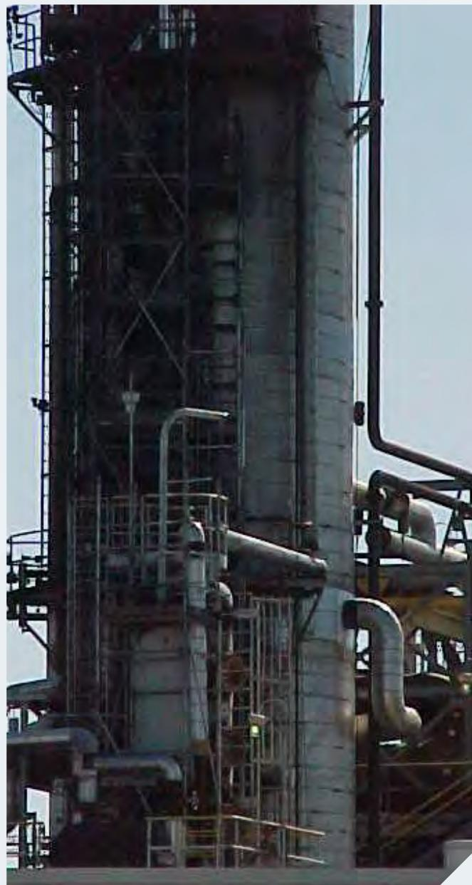
processed excessive volumes of crude oil with high water content, overtaxing the desalter. As a result, water and corrosive materials, like ammonium chloride, were carried over into the fractionator, where they deteriorated the piping and valves.
