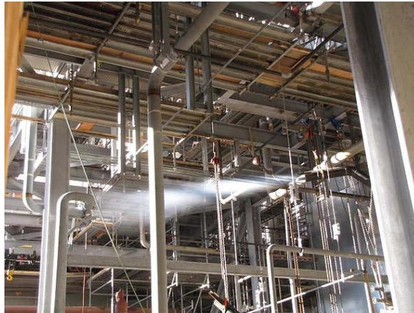
This cleaning practice is known within the natural gas power industry as a “gas blow.” Industry personnel have indicated to CSB investigators that gas blows are a common practice during the commissioning of new or modified gas pipes at their facilities.
