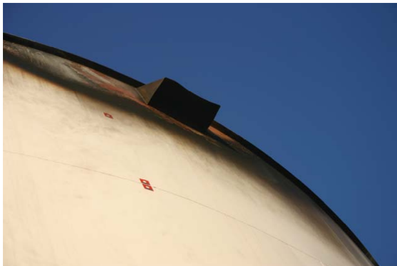
Atmospheric vent on roof of Tank 105.
