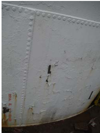
E. SHELL COATING FAILURE ALONG EXTERIOR SHELL
