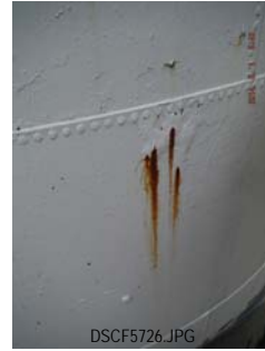
COATING FAILURE AND CORROSION ALONG SHELL PLATES
