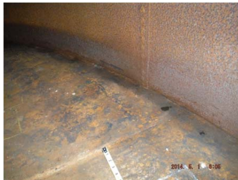
Photo of typical crack location
