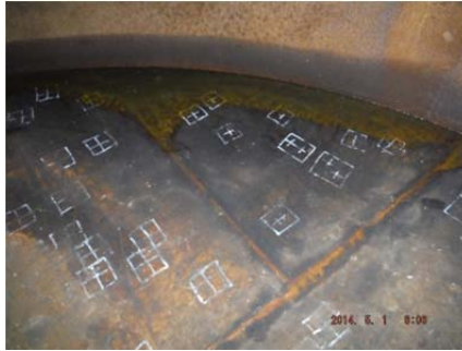
MFE Bottom Indication Marks (Immediately after marking)
