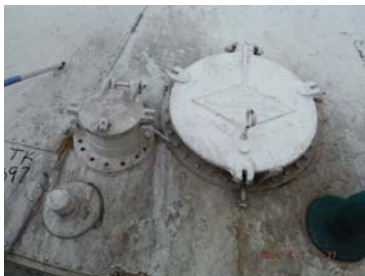
CORROSION ALONG THE ROOF DECK
