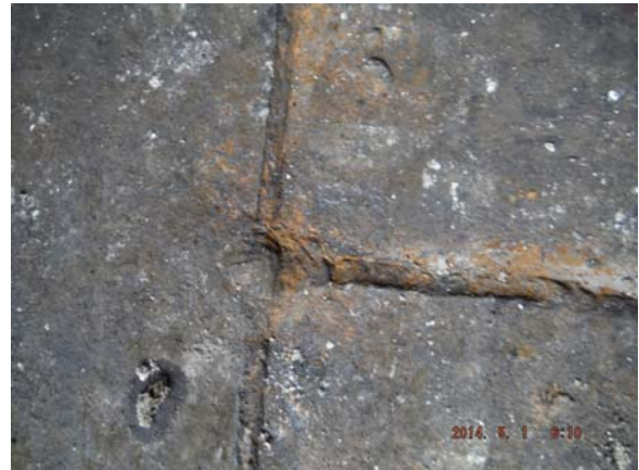
F. BOTTOM PITTING ALONG BOTTOM PLATES
