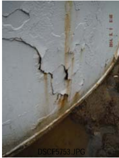
COATING FAILURE AND CORROSION ALONG SHELL PLATES
