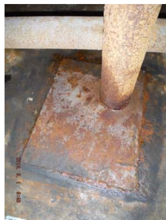
F. BOTTOM REPAD NOT SEAL-WELDED TO BOTTOM: COUND NOT INSPECT UNDERNEATH
