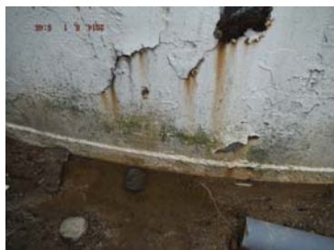
WATER IN CONTACT WITH BOTTOM PLATES
