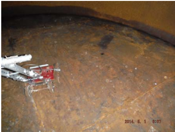
F. BOTTOM WATER AND DIRT PREVENTED ACCURATE UT PROVE-UP OF MFL INDICATIONS
