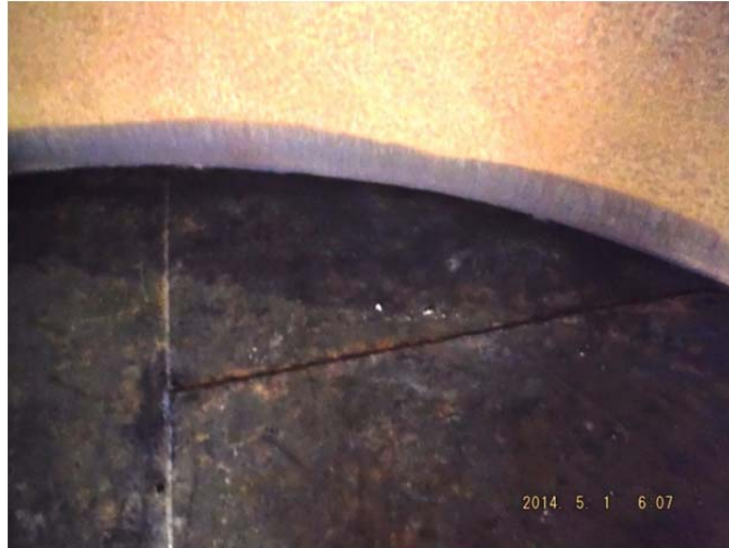
Typical Bottom Lap Weld
