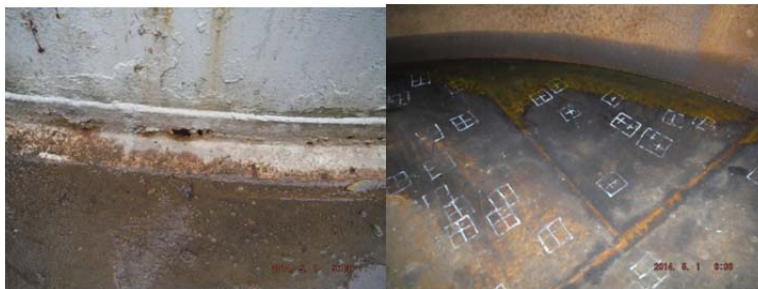
Muddy Conditions around the base of the tank and debris inside tank
