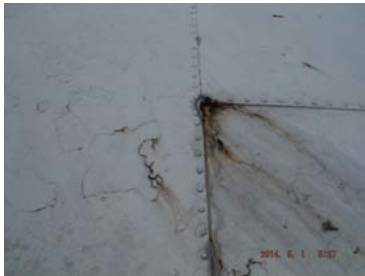
CORROSION ALONG THE ROOF DECK
