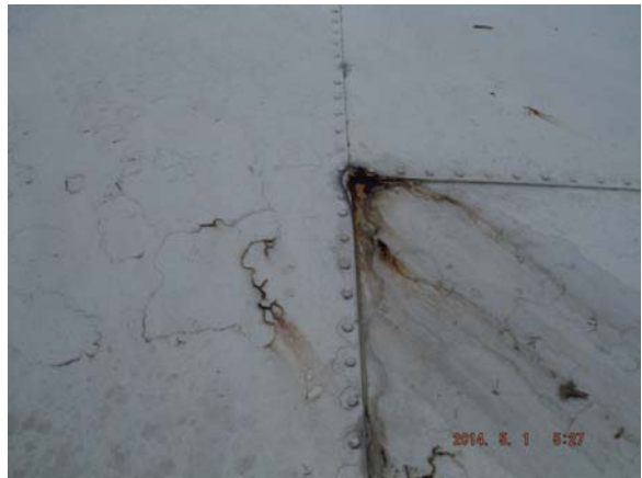
D. ROOF CORROSION ALONG THE ROOF DECK
