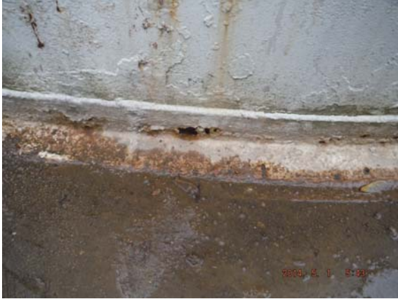
B. FOUNDATION COATING FAILURE ALONG THE BOTTOM ANGLE
