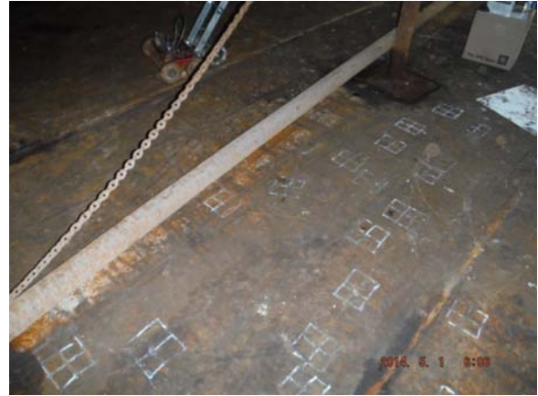
F. BOTTOM WIDE SPREAD MFL INDICATIONS OF SOIL-SIDE CORROSION
