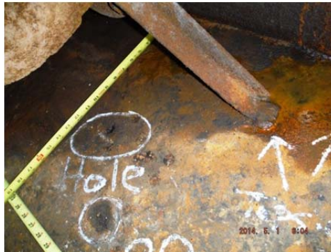
Hole on bottom from product side pitting
