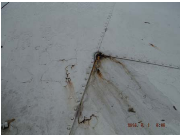
D. ROOF COATING FAILURE AND CORROSION ALONG ROOF DECK
