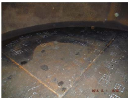
Bottom Conditions at Time of Inspection
