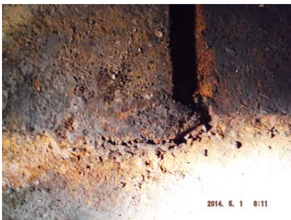
F. BOTTOM PRODUCT-SIDE CORROSION ALONG BOTTOM PLATES
