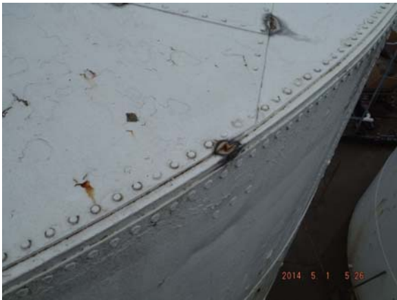
D. ROOF COATING FAILURE AND CORROSION ALONG UPPER ANGLE
