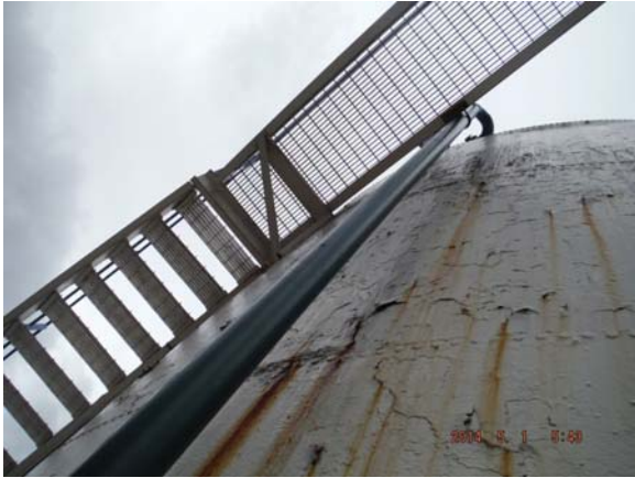
E. SHELL COATING FAILURE ALONG THE SHELL
