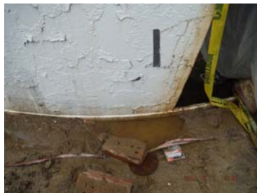
WATER IN CONTACT WITH BOTTOM PLATES
