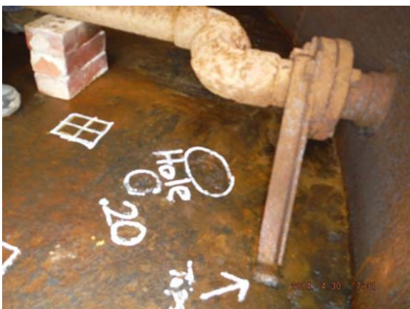
F. BOTTOM 0.200-IN PITTING AND THROUGH HOLE CORROSION ON THE BOTTOM PLATES
