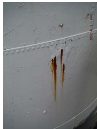
E. SHELL COATING FAILURE AND CORROSION ALONG SHELL PLATES
