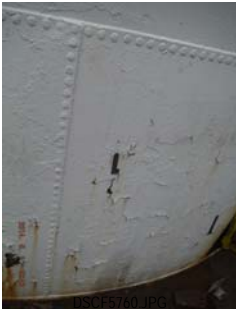
COATING FAILURE ALONG EXTERIOR SHELL
