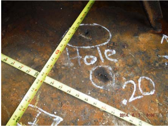
F. BOTTOM THROUGH-HOLE CORROSION AND 0.200-IN DEEP PITTING ALONG BOTTOM PLATES
