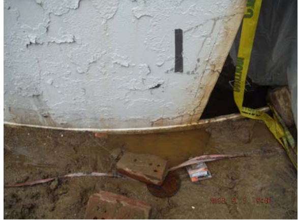
B. FOUNDATION WATER IN CONTACT WITH BOTTOM PLATES
