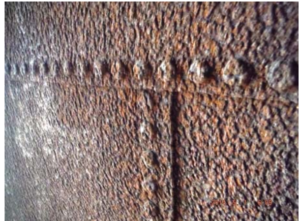
E. SHELL CORROSION ALONG THE INTERIOR SHELL PLATES
