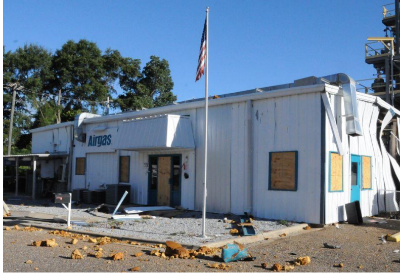
Figure 2. Post-incident photo of the administrative and operations building at the Airgas nitrous oxide manufacturing facility in Cantonment, Florida nitrous oxide manufacturing facility. Although the official corporate name is Nitrous Oxide Corp., the Airgas name is more commonly used.
