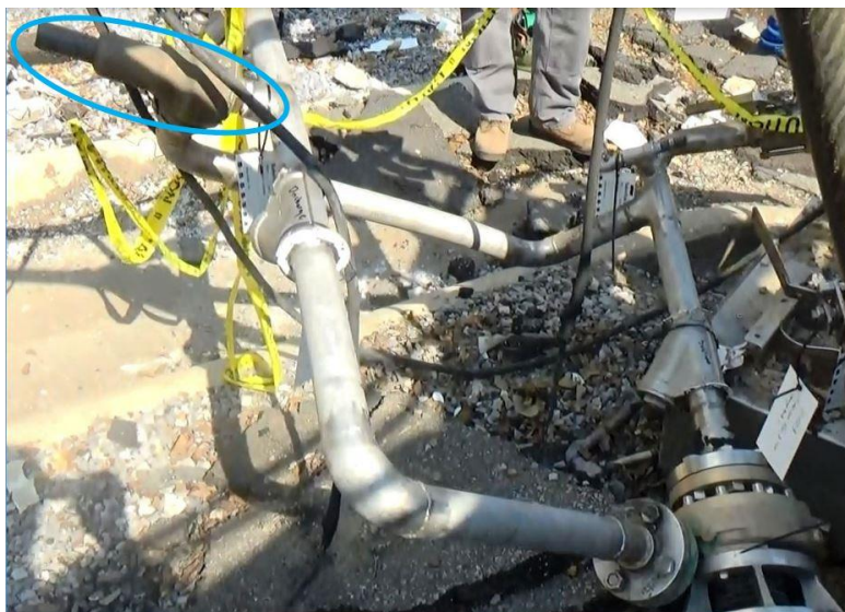
Figure 39. Photo of the ACD pump relief valve (blue oval). Post-incident testing showed that this valve likely circulated nitrous oxide back to the pump inlet. Due to the low temperature of the nitrous oxide (about -10 °F), this piping is insulated. This photo shows the piping after removal of the insulation.
