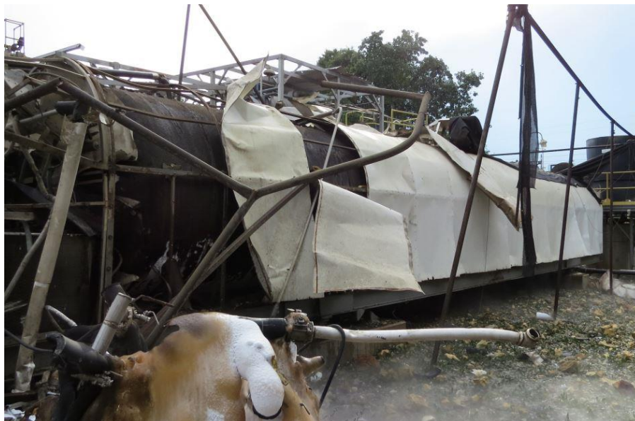
Figure 4. Post-incident photo showing one of the three 50-ton nitrous oxide storage tanks.
