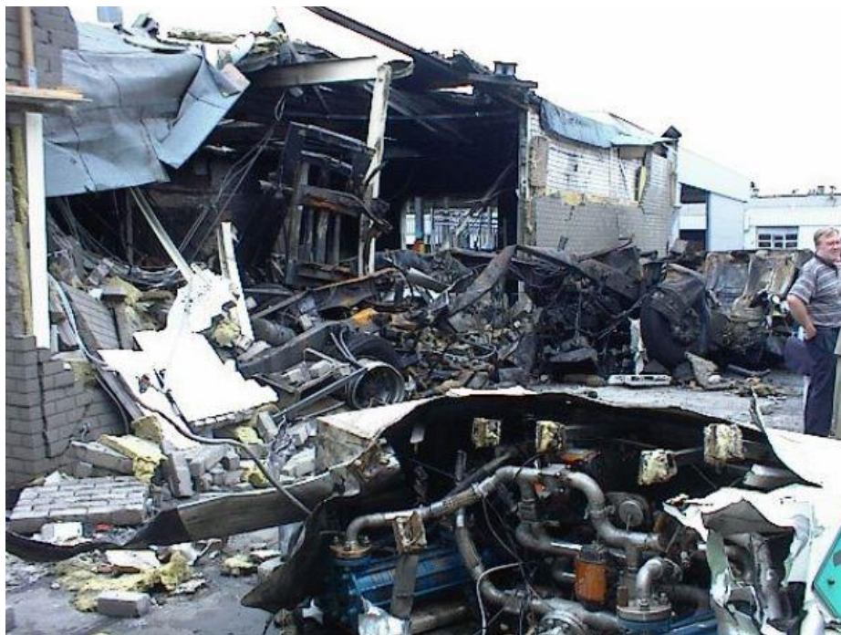
Figure 13. Photo of damage following the July 2001 nitrous oxide truck-filling explosion in Eindhoven, the Netherlands. Photo from [1]. 79
