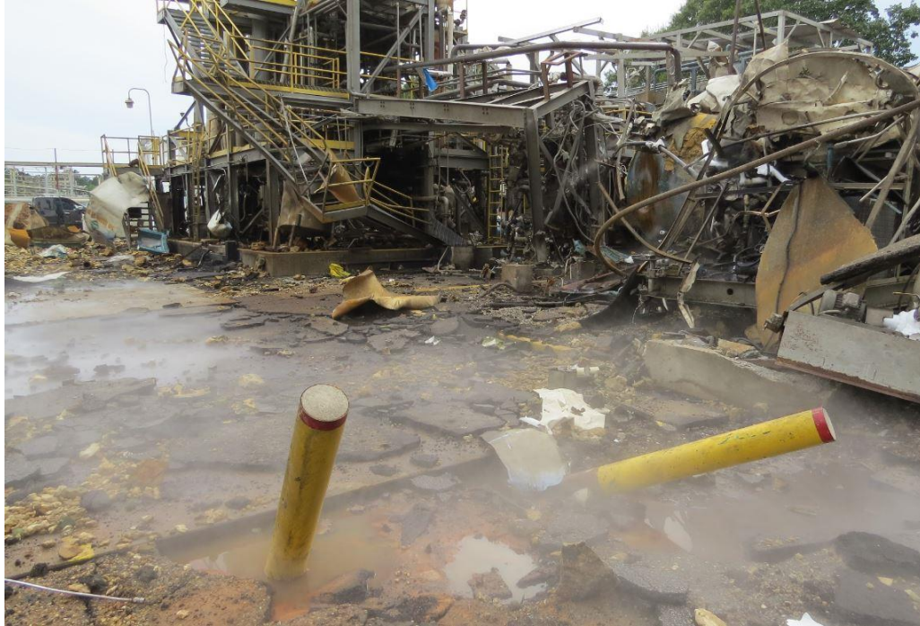
Figure 18. Photo showing explosion damage at the Airgas facility in Cantonment, Florida.
