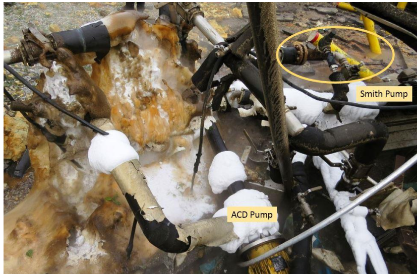
Figure 38. Post-incident photo showing the ACD pump inlet and outlet piping to the trailer loading piping. The explosion breached the discharge piping system and drained the remaining nitrous oxide in the storage tank to atmosphere. The frost line on the equipment shows this flow exited through the ACD pump. The discharge of the Smith pump (yellow oval) is not frosted and the discharge valve is closed.
