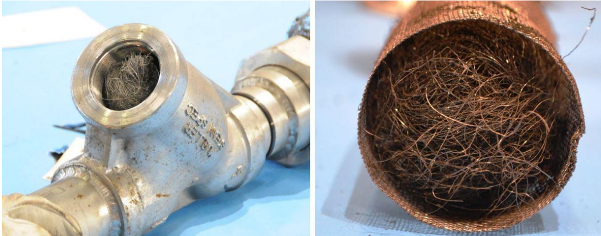
Figure 30. Airgas uses strainers filled with steel wool on pump suction and discharge piping to serve as a flame arrester. Airgas relies on these strainers to prevent a nitrous oxide decomposition reaction from propagating to the trailer being filled, where the reaction could result in an explosion. The left photo shows a y-strainer recovered from the Cantonment site with its cap removed revealing the basket filled with steel wool. The right photo shows a close-up of a different y-strainer basket also recovered from the Cantonment site containing steel wool.
