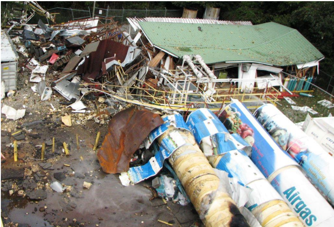
Figure 21. Post-incident photo that shows damage from the explosion. Trailer 182 and Trailer Y-3 were originally located in the lower left quadrant of this photo.
