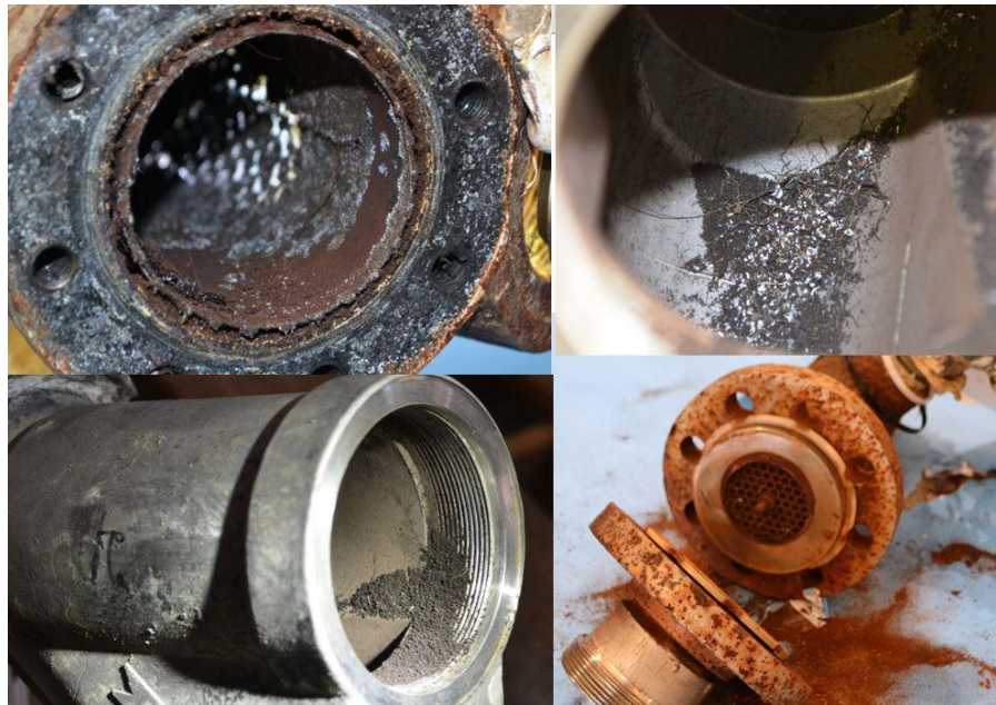
Figure 46. Photos of strainer corrosion and metallic particles. Post-incident evaluation of nitrous oxide pump strainers revealed equipment corrosion and metallic particles. These metallic particles may have acted as a contaminant and could have played a role in the explosive nitrous oxide decomposition reaction.
