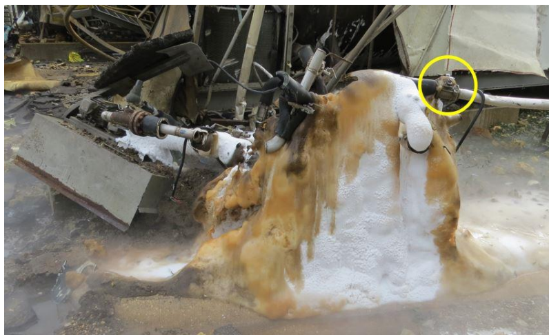
Figure 51. Post-incident photo of the nitrous oxide transfer pumps. The yellow circle identifies the nearly closed discharge valve – a quarter-turn ball valve.
