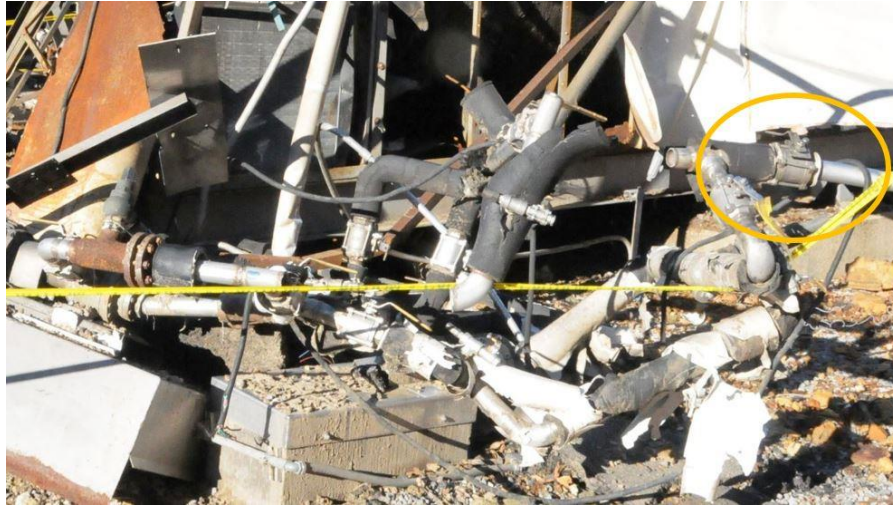
Figure 52. Post-incident photo of nitrous oxide transfer pumps. The orange oval shows the discharge valve that may have nearly closed during the explosion by the Trailer 182 power cable. The open position of this valve handle is towards the left and parallel to the piping. This is the same valve circled in yellow in Figure 51
