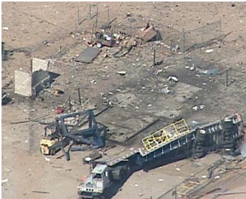
Figure 14. Photo of damage following the July 2007 nitrous oxide tank explosion in Mojave, California. Photo from parabolicarc.com 84
