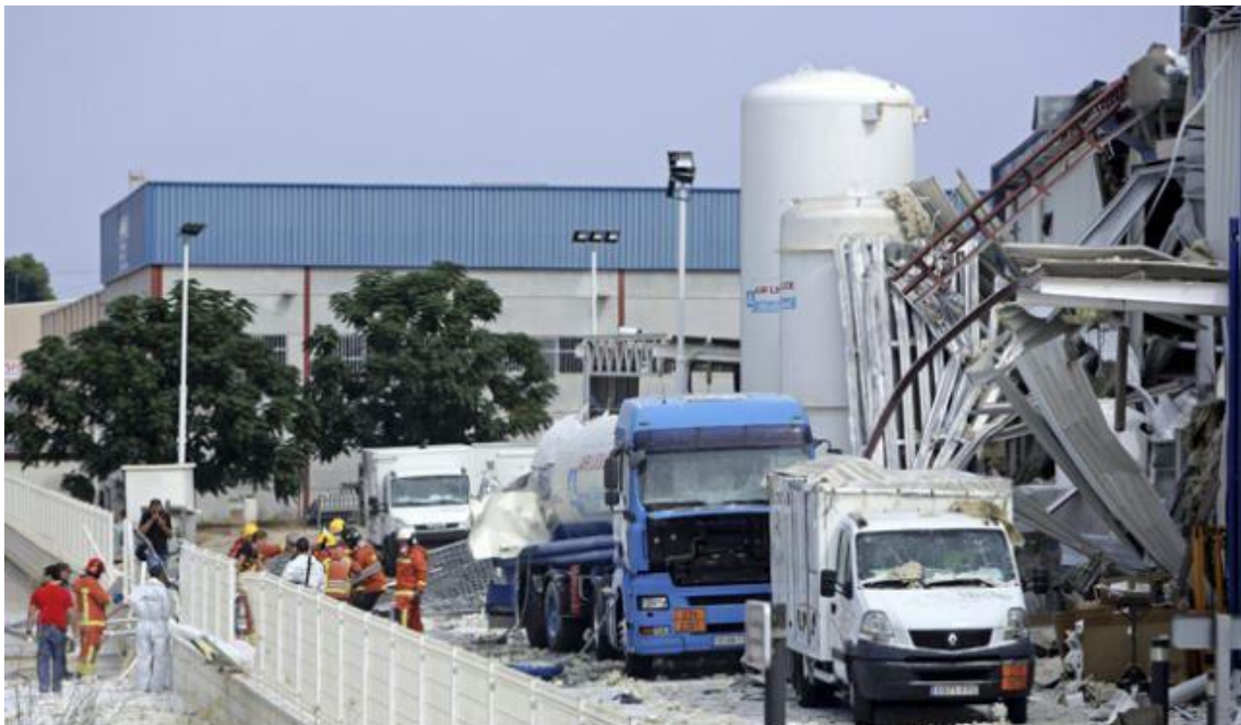
Figure 15. Photo of the damage following the September 2012 nitrous oxide explosion in Moncada, Spain. 99
