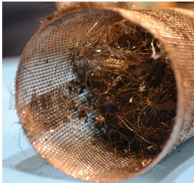
Figure 35. Photo showing the top end of the ACD pump suction piping y-strainer basket with missing and discolored steel wool.
