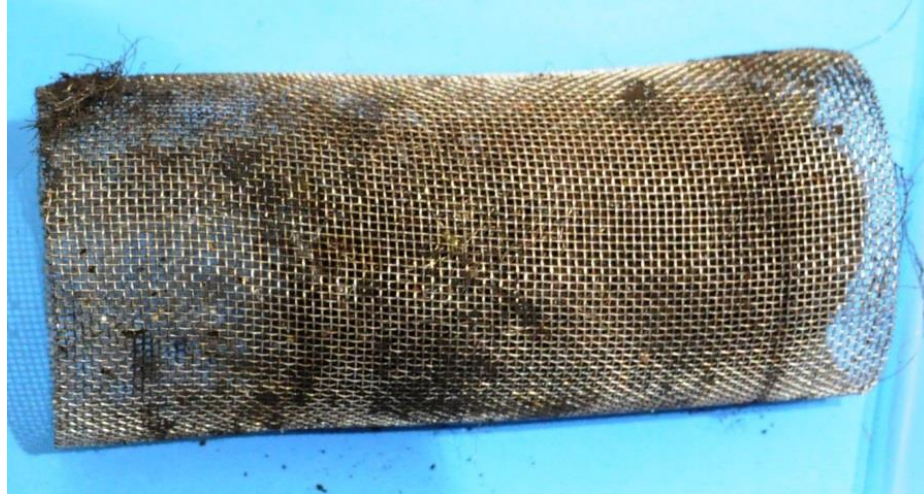
Figure 34. Photo of y-strainer basket from the inlet piping to the ACD pump. The left side of the basket is inserted the furthest into the y-strainer.
