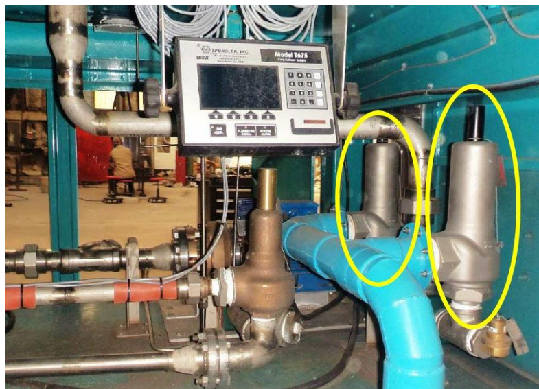
Figure 49. Trailer 182 relief valves. This pre-incident photo taken at a maintenance facility shows the location of the two relief valves (yellow ovals) that protect Trailer 182 from high pressure. Only one valve is in service at a time. A 3-way valve, obscured by the blue piping, can change which valve is in service.
