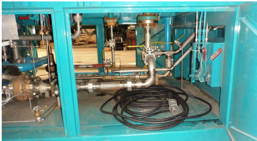
Figure 53. Pre-incident photo of the black electrical cable located inside the equipment box located at the bottom and towards the rear of Trailer 182. This photo also shows an example of the flexible hose connections recommended by pump manufacturers and used by Airgas on trailer pumps.
