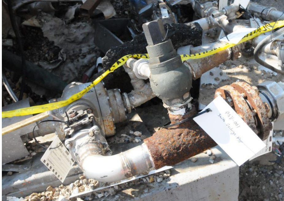
Figure 59. Photo of the Smith nitrous oxide pump discharge piping. From the outlet of this positive displacement pump, there is an isolation block valve upstream of the relief valve. As a result, the equipment may not be adequately protected from a scenario where this isolation valve was inadvertently closed while operating the pump.
