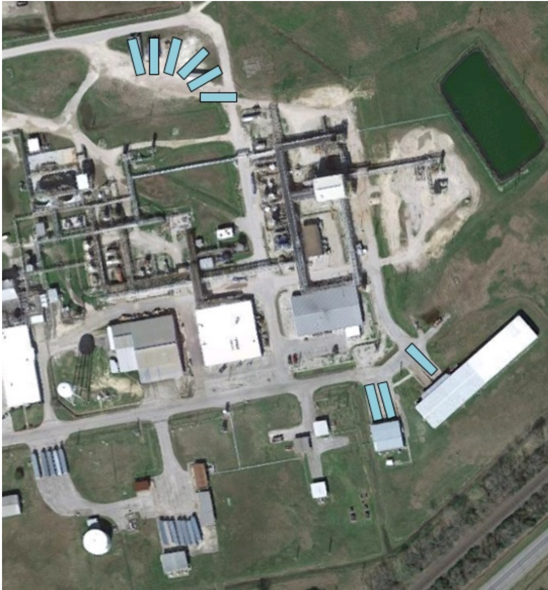
Figure 27. Location of the Nine Refrigerated Trailers Containing Organic Peroxide Products. (Source: Google Earth Image Modified by CSB)
