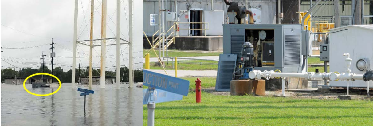
Figure 19. One of the Emergency Generators Providing Backup Electricity to the Low Temperature Warehouses. The photo on the left shows floodwater covering the bottom half of the generator (yellow oval) on Tuesday August 29, 2017. The post-incident photo on the right shows the same generator. (Source: Arkema Photo (left) Modified by CSB, CSB Photo (right))
