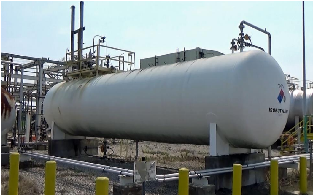
Figure 43. Isobutylene Storage Tank at the Arkema Crosby Facility. The isobutylene tank posed a concern because the controlled burn of the six refrigerated trailers in the laydown area would occur within about 40 yards of this storage tank. (Source: CSB Photo)
