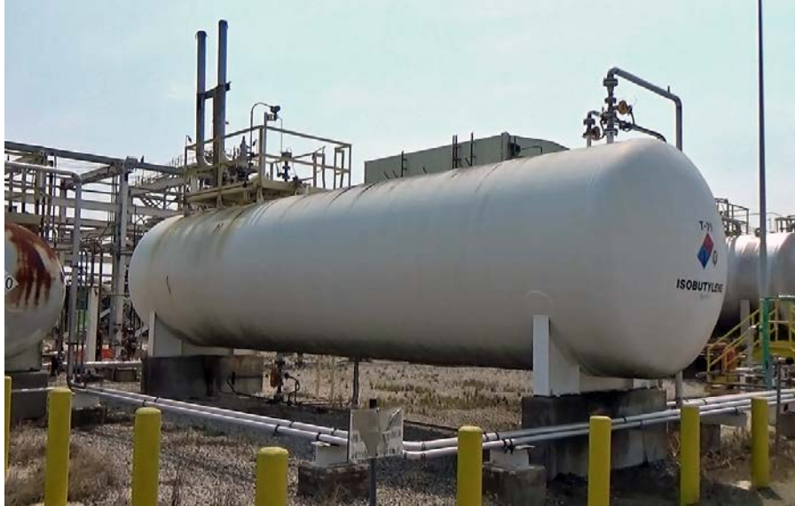
Figure 59. Arkema Crosby Isobutylene Storage Tank. The isobutylene storage tank at the Arkema Crosby facility was located more than 100 feet from the nearest refrigerated trailer containing organic peroxide products. (Source: CSB Photo)
