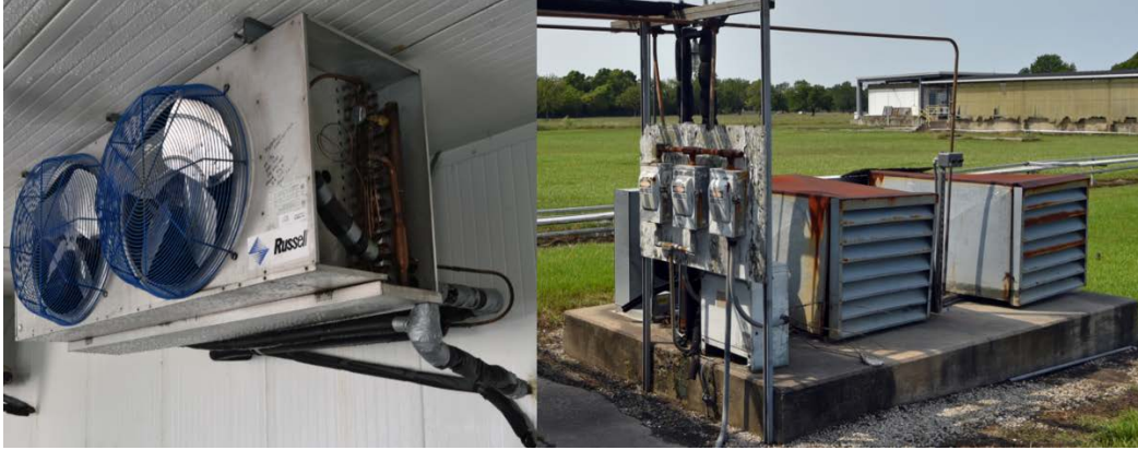
Figure 4. Typical Refrigeration Equipment Used to Keep the Low Temperature Warehouses Cold at the Arkema Crosby Facility. The photo on the left shows refrigeration evaporator equipment used to remove heat from the inside of a Low Temperature Warehouse. The photo on the right shows refrigeration condensing equipment, that removes heat from the refrigerant and also shows electrical equipment for the refrigeration system and other electrically powered equipment for the building, such as lighting. a (Source: CSB Photo)
