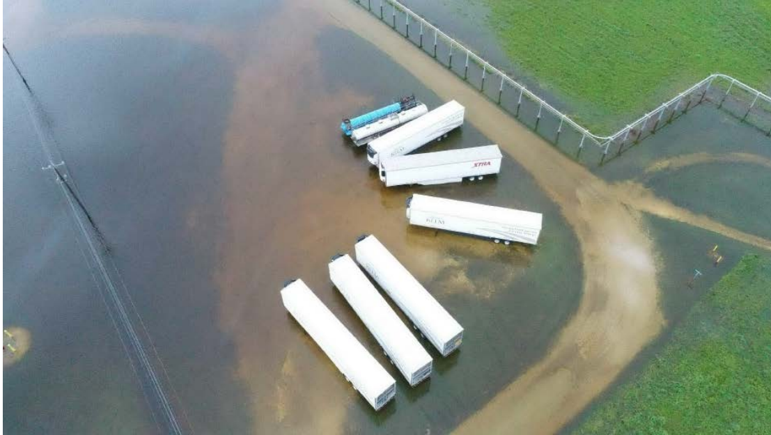
Figure 21. Refrigerated Trailers in the Laydown Area. Six refrigerated trailers loaded with organic peroxide products are shown at the Arkema Crosby facility. Two empty tanker trailers are also shown at the top of the photo. (Source: Photo provided by Arkema)
