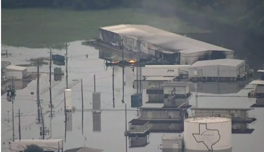
Figure 39. First Refrigerated Trailer to Burn at the Arkema Crosby Facility. The first refrigerated trailer to burn is shown smoldering outside of Building 21 [37].
