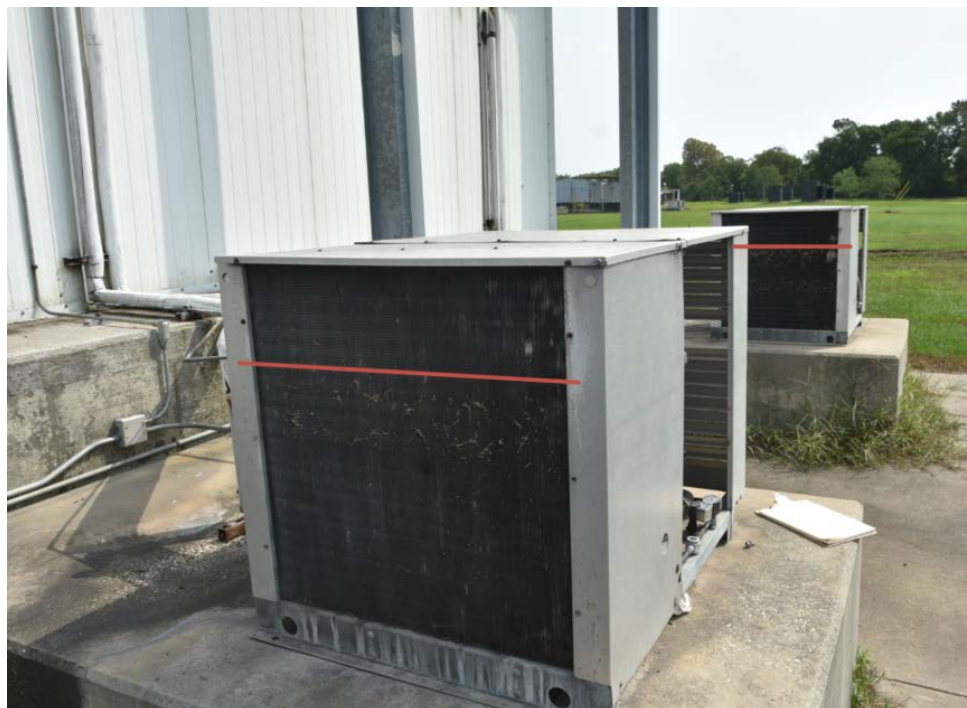
Figure 17. Air Conditioning Units Behind One of the Low Temperature Warehouses. The final floodwater level is approximated by the red lines on the air conditioning equipment at the Arkema Crosby facility. (Source: CSB Photo)
