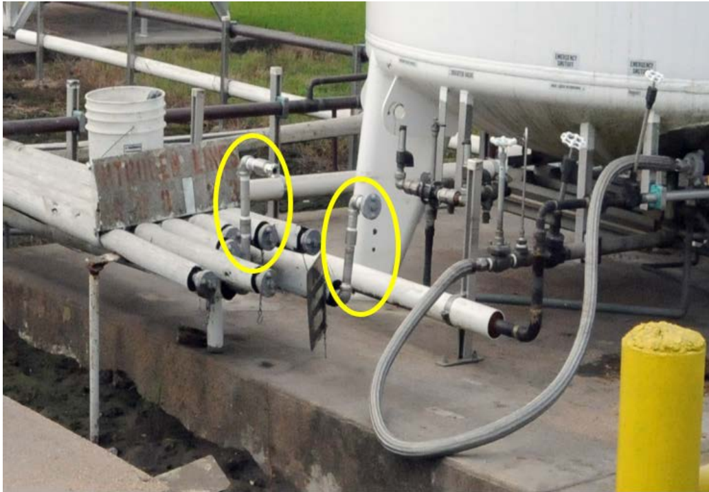
Figure 20. Liquid Nitrogen Piping Extensions. A supervisor modified the liquid nitrogen piping, extending it to ensure that the connection point would be above the floodwater if the ride-out crew needed to inject liquid nitrogen into one of the Low Temperature Warehouses that still contained organic peroxide products. These elevated (extended) connections, however, were not high enough; the rising floodwater eventually submerged them. (Source: CSB Photo)
