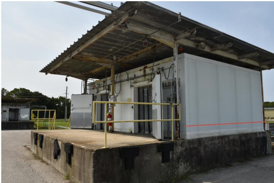
Figure 29. Low Temperature Warehouse at the Crosby facility. The red line shows the high-water mark, just over five feet above the ground. (Source: CSB Photo)
