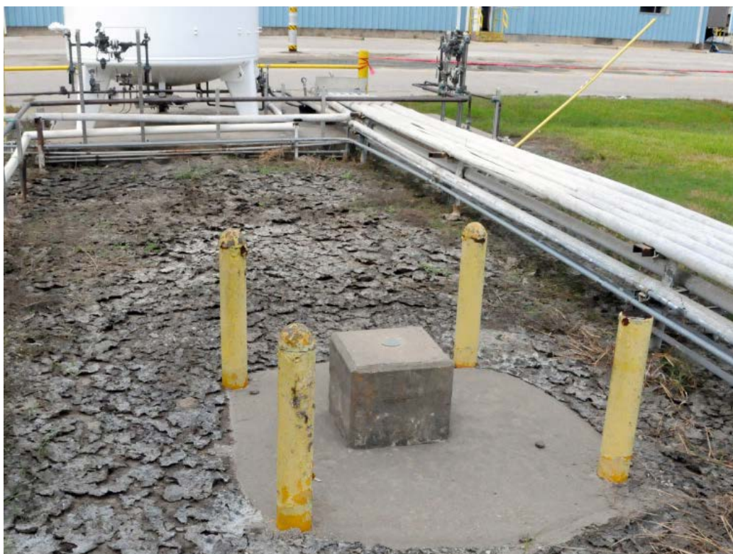
Figure 55. Elevation Survey Marker Near the Liquid Nitrogen Storage Tank. The metal plate on top of the concrete block shows that the elevation is 51.5 feet, about six inches lower than the base flood elevation. During Hurricane Harvey, floodwater exceeded the height of the survey marker by more than three feet. (Source: CSB Photo)
