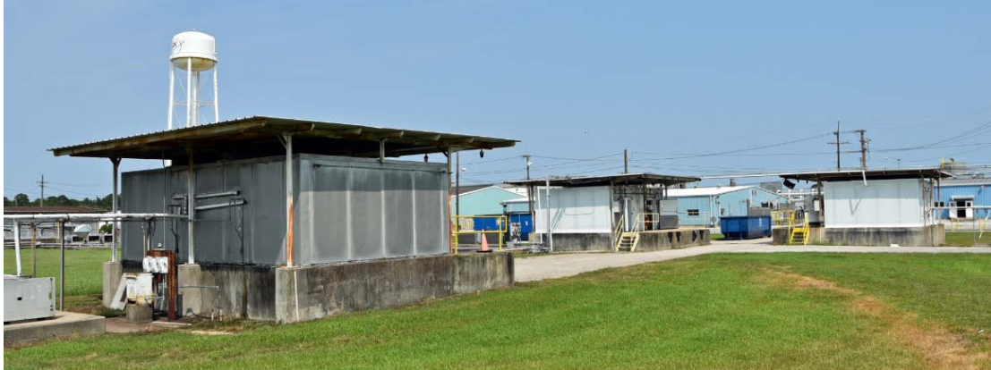
Figure 3. Crosby Low Temperature Warehouses. Three of the seven Low Temperature Warehouses at the Arkema Crosby facility are shown in this photograph. (Source: CSB Photo)
