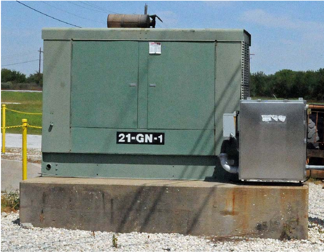
Figure 5. One of Seven Emergency Generators at the Arkema Crosby Facility. Generator 21-GN-1 is one of the two generators providing emergency electrical power to Arkema's seven Low Temperature Warehouses. The bottom of the generator (top of the concrete foundation) is about two feet above the ground. (Source: CSB Photo)
