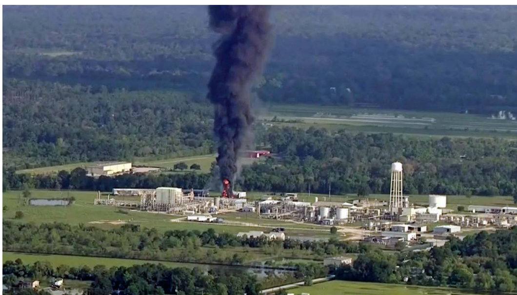
Figure 40. The Second and Third Refrigerated Trailers Burning. Fire and smoke are visible from two refrigerated trailers burning at the Arkema Crosby facility on September 1, 2017 [40].
