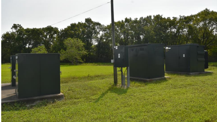
Figure 24. CenterPoint Transformers at the Arkema Crosby Facility. These are the main CenterPoint power transformers onsite at the Arkema Crosby facility. (Source: CSB Photo)
