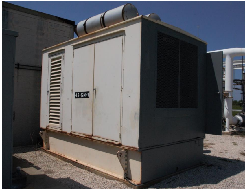
Figure 25. Emergency Generator. This is one of the emergency generators that automatically turned on when the power failed at the Arkema Crosby facility. (Source: CSB Photo)
