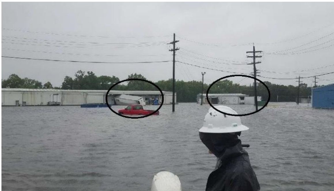
Figure 31. Condition of the Crosby Facility on the Morning of Tuesday, August 29, 2017. The ride-out crew sent this photograph to the corporate crisis team showing the trailer on the left had tilted. (Source: Arkema Photo Modified by CSB)
