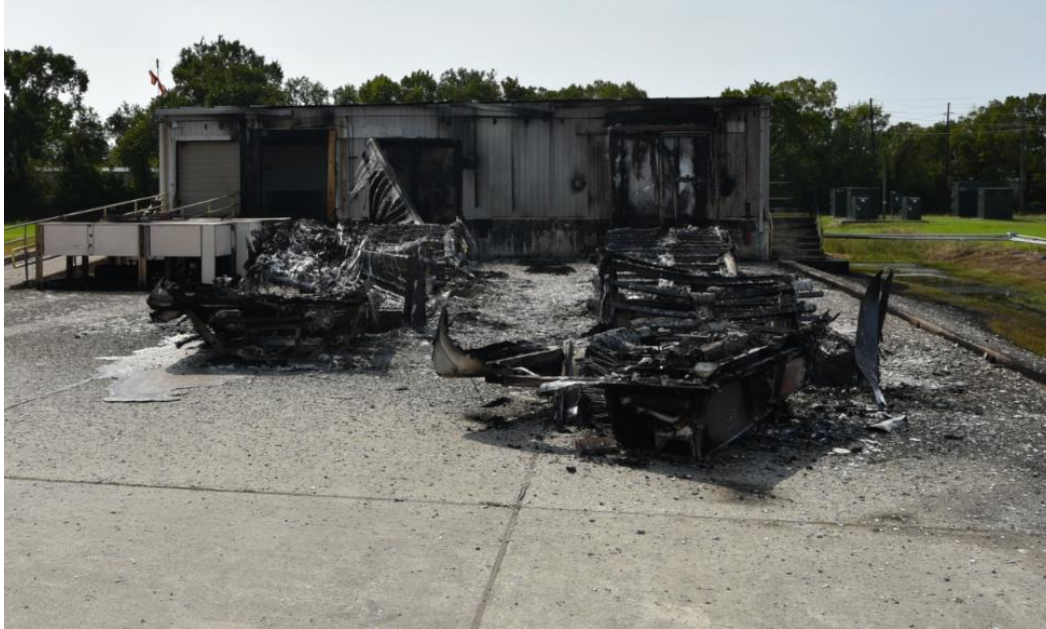
Figure 41. Remains of the Second Fire that Consumed Two Trailers Storing Organic Peroxide Products. The second fire consumed two refrigerated trailers storing organic peroxide products; the remains of those trailers are shown in this image. (Source: CSB Photo)
