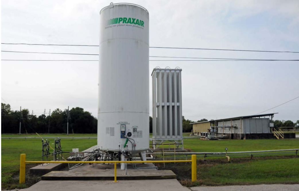
Figure 6. Liquid Nitrogen Tank at the Arkema Crosby Facility. Among other uses, this tank holds up to 40,000 pounds of liquid nitrogen that can be injected into each of the organic peroxide Low Temperature Warehouses to provide a backup refrigeration source. (Source: CSB Photo)
