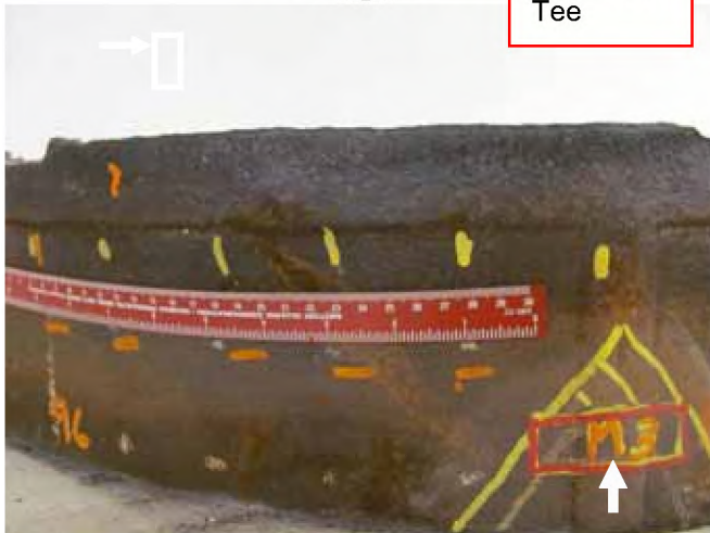
Looking at OD surface CS4 top with LS4 the vertical weld at the Tee into CS4
