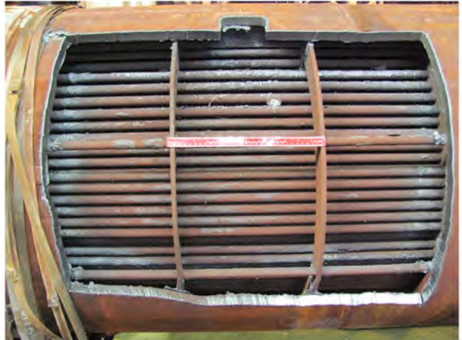
Cut out of shell
