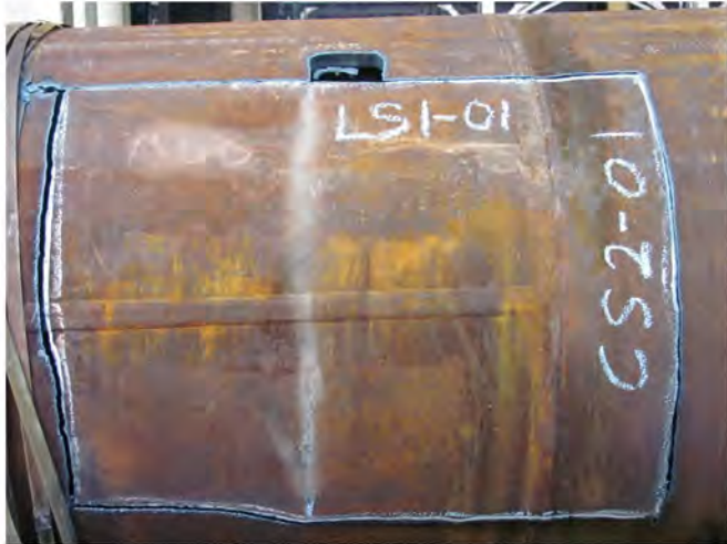
Cut ready for removal
