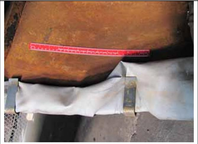
Fracture protection blankets and clip attachments
