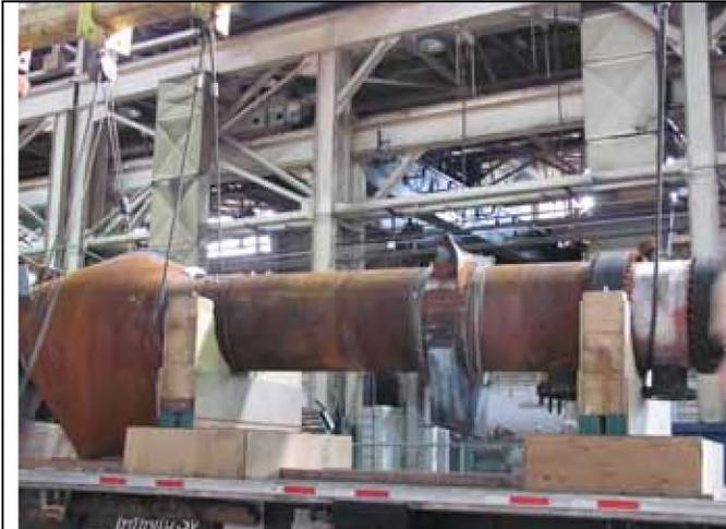
Main hear exchanger stripped of plastic sheets and rigged for lifting
