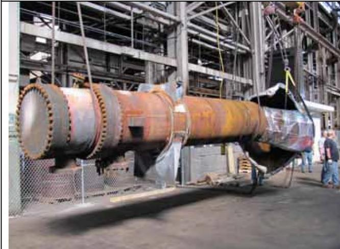
Main heat exchanger ready for wood saddle support insertion
