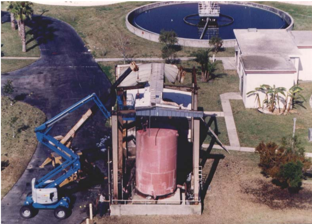
Figure 2. Bethune Point WWTP accident site.
