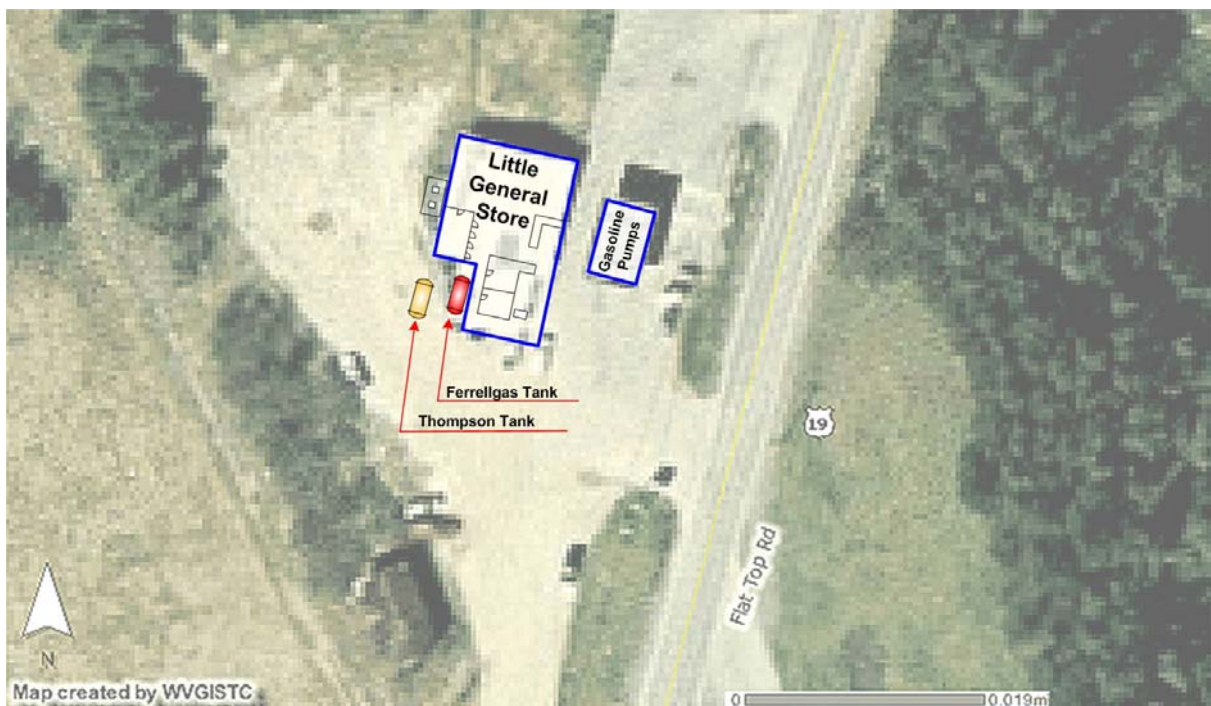
Figure 1. Aerial photograph of Little General store and surrounding plot.
