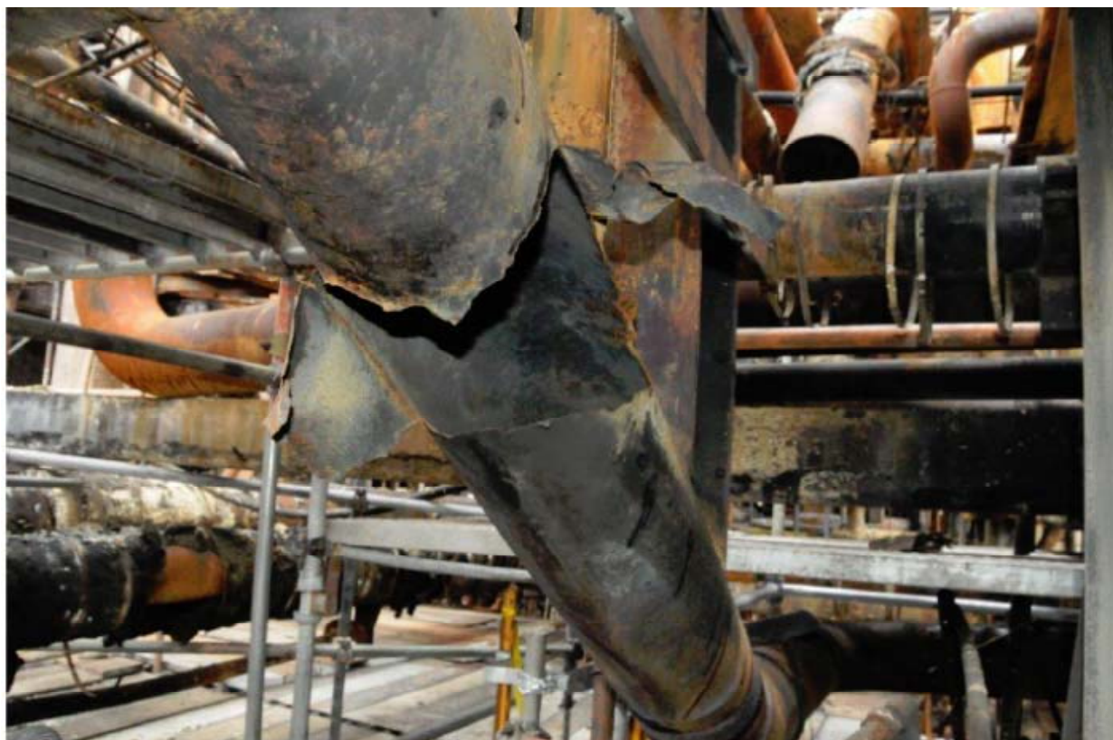
Figure 5. Photo of rupture on 4-sidecut 52-inch component.
