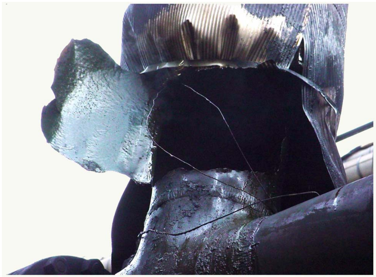
Figure 38. Photo from API RP 939-C of a low-silicon pup piece that ruptured at a BP refinery. The surrounding piping had higher silicon content, and the pup piece’s accelerated corrosion rate was unmonitored.
