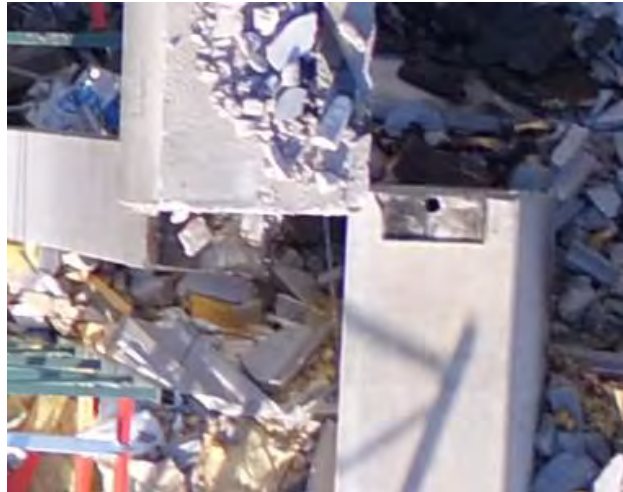
Figure 2-16. Multipurpose Building Beam Grout Hole
