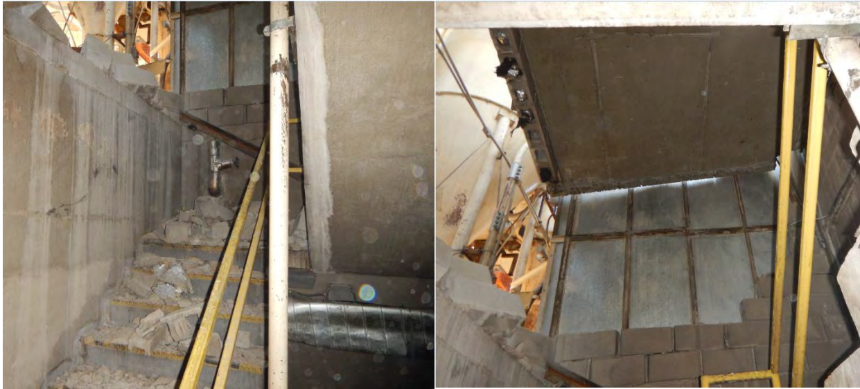
Figure 3-24. Mill A Level 6 Access
