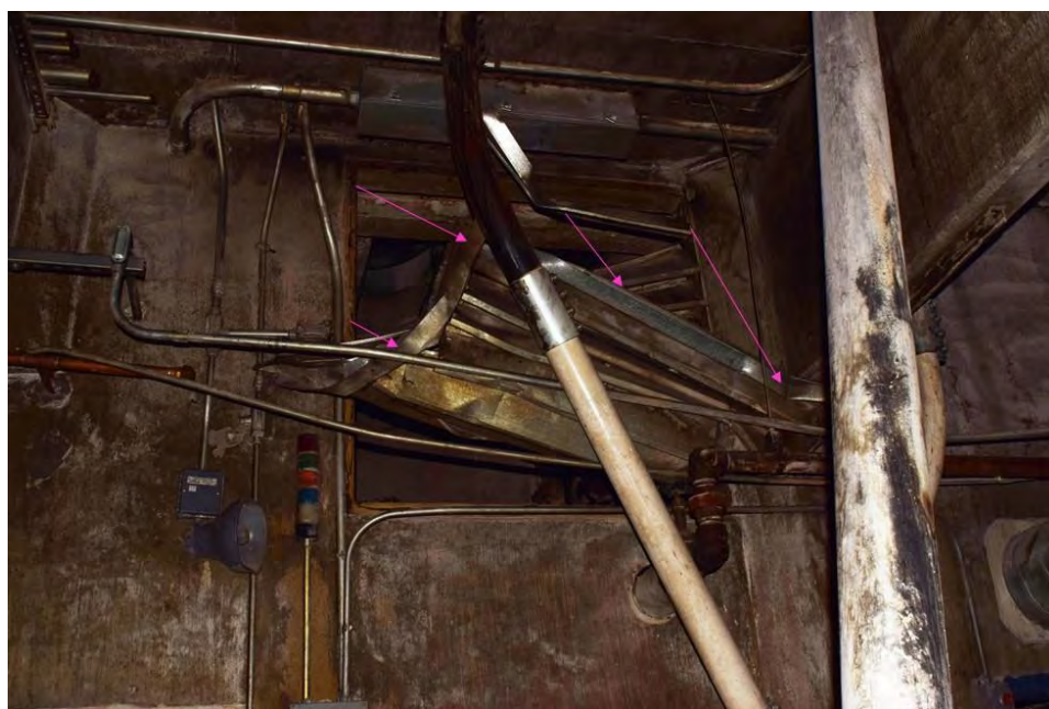
Figure 3-23. Mill A Level 5 Air Shaft Opening Directional Indicator
