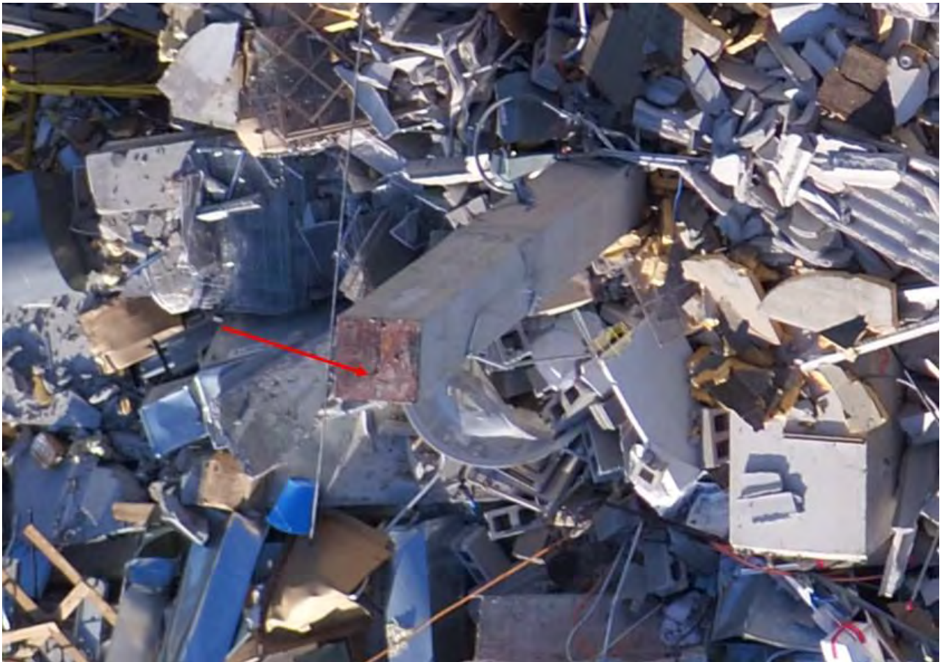
Figure 2-17. Multipurpose Building Top of Column with Visible Dowel
