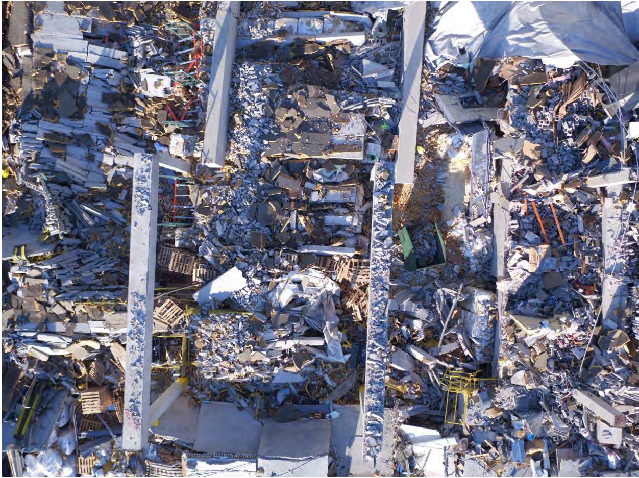
Figure 2-19. Top of Multipurpose Building Beams
