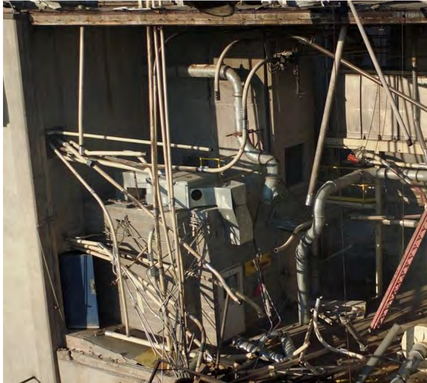
Figure 3-20. Mill B Level 4 Air Shaft Opening
