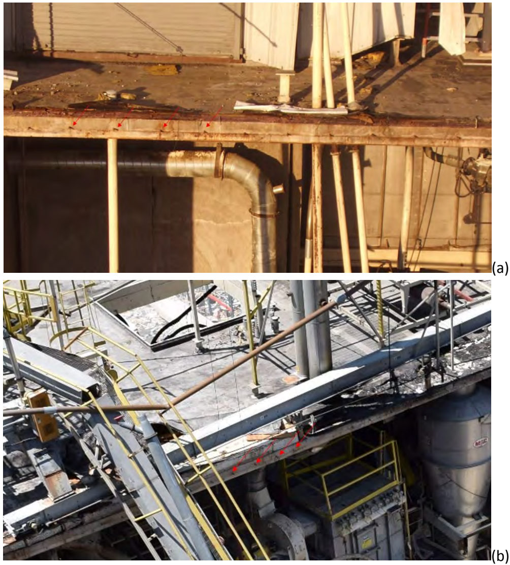
Figure 2-10. Mill B Wall Panel Roof Slab (a) West Façade (b) East Façade
