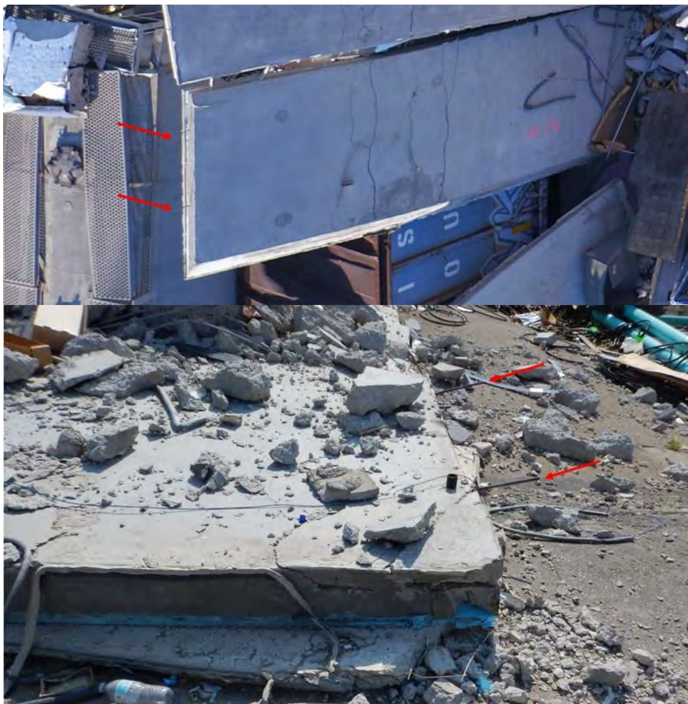
Figure 2-21. Multipurpose Building Load Bearing Wall Dowels into Hollow Core Planks
