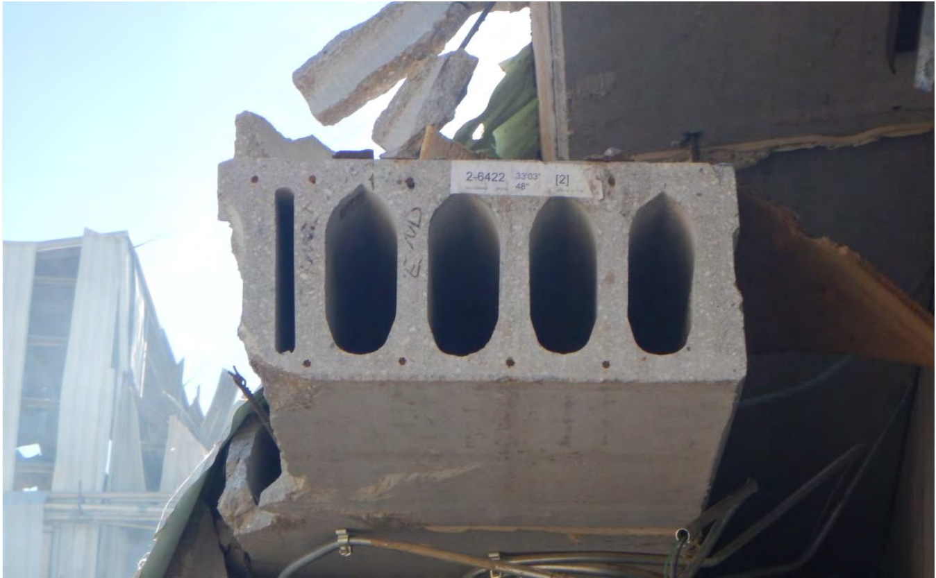
Figure 2-13. Multipurpose Building Hollow Core Roof Plank
