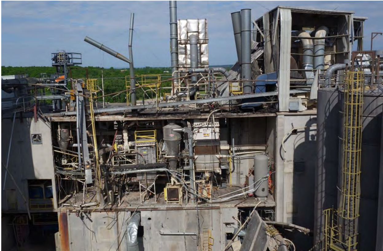
Figure 2-7. Mill B East Façade at 4 th Level
