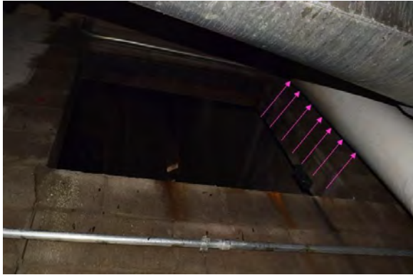
Figure 3-16. Mill B Level 3 Air Shaft Opening Fire Directional Indicator
