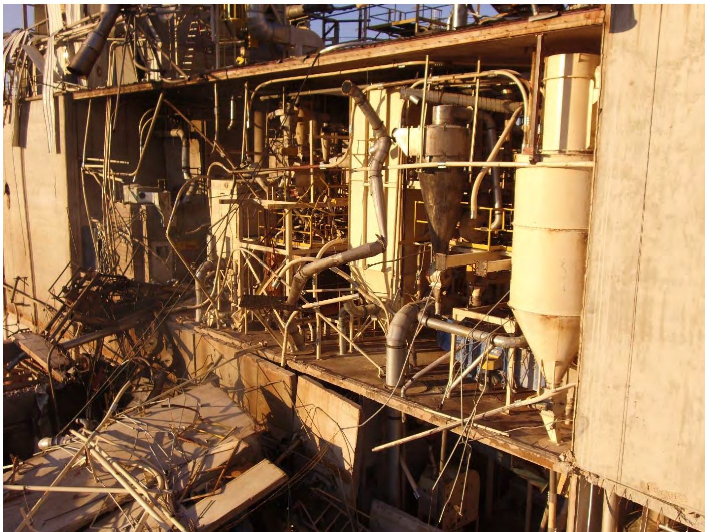
Figure 2-6. Mill B West Façade at 4 th Level
