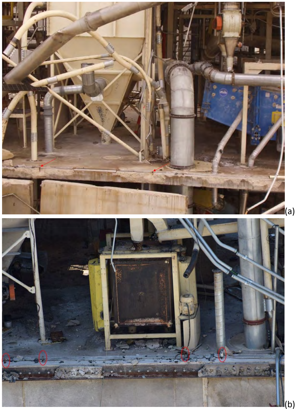
Figure 2-9. Mill B Wall Panel Bottom Connection at 4 th Level (a) West Façade (b) East Façade
