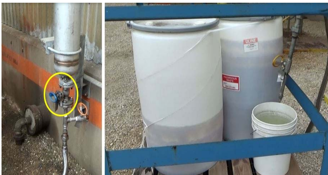
Figure 37. Photo Showing Another Line Break. Operators drained liquid accumulation in another vent header without using line-breaking procedures. Source: CSB.
