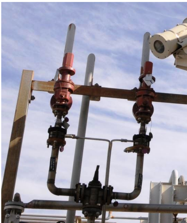
Figure 33. Nitrogen Relief Valves at One of the Two Methyl Mercaptan Railcar Unloading Stations. DuPont PHAs and relief valve design documents never considered the possibility of lining up the methyl mercaptan storage tank pumps to these relief valves—as they were at the time of the incident. As a result, liquid methyl mercaptan was discharged from a system designed for nitrogen vapor. Source: CSB.
