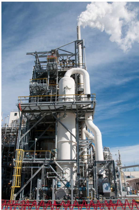
Figure 34. NRS Incinerator. NRS was installed in 2011 to reduce emissions and allow increased production at the DuPont La Porte facility. Source: CSB.
