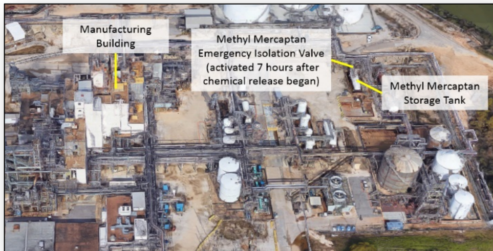
Figure 13. Location of Methyl Mercaptan Emergency Isolation Valve Relative to Manufacturing Building Where Leak Occurred. The emergency isolation valve was not activated until seven hours after the release began. Source: Google Earth, with annotations by CSB.
