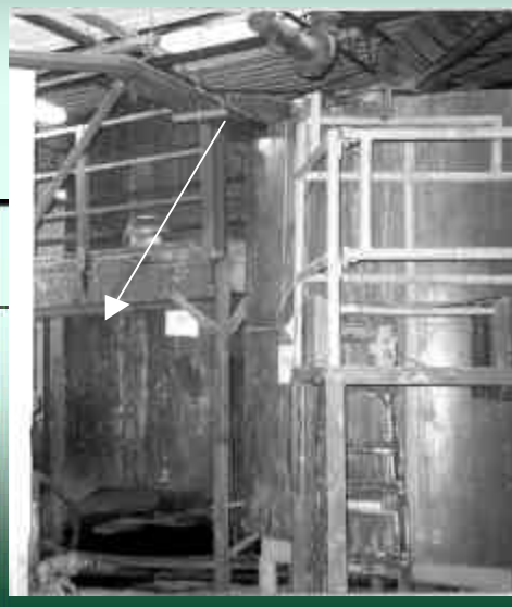
Figure 1 Open-top WWT clarifier
