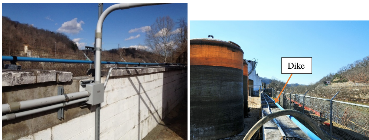
Figure 23. View from inside the dike wall facing the Elk River of the concrete block walls with no reinforcement (Left); dike wall along the tank farm parallel to the Elk River (Right). (Source: CSB)
