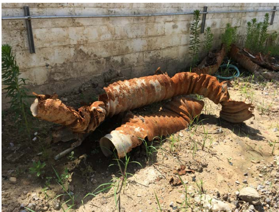
Figure 28. Photo taken on June 15, 2015, of remnants of the culvert that ran between tanks 394 and 395 beneath the site. (Source: CSB)
