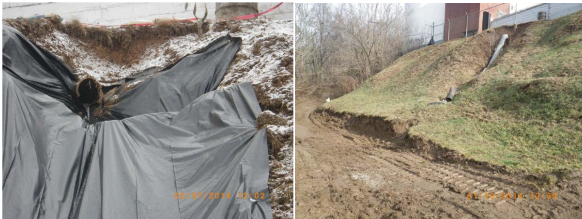
Figure 27. Water flowing through a corrugated steel culvert extending from the hillside (Left); stormwater pipe above interceptor trench (Right). (Source: WVDEP)
