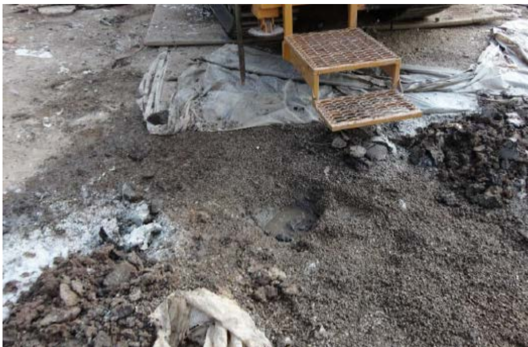
Figure 20. Gravel base under tank 396 and other tanks containing mixtures with Crude MCHM and PPH, Stripped. (Source: Terracon)
