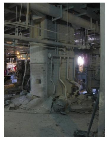
This photograph shows the reflux tower after the explosion. The trays in the combustion chamber have collapsed but the reflux tower is largely undamaged, having dropped a few feet such that the framework for the reflux section insulation was sitting on the combustion chamber roof.
